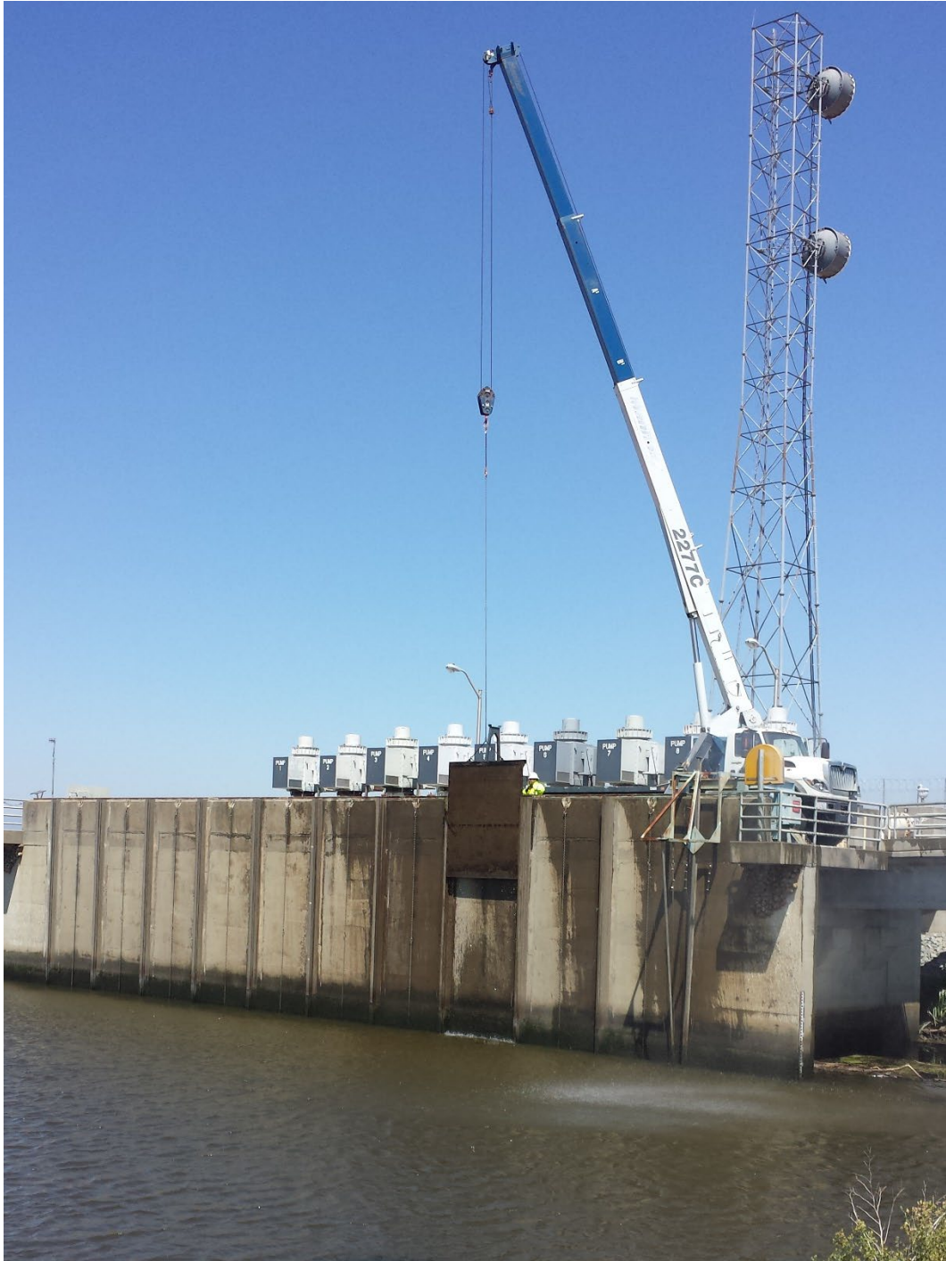
Exhibit 6. Photo of Crane and Hook Used to Lift Fish Screens for Cleaning
