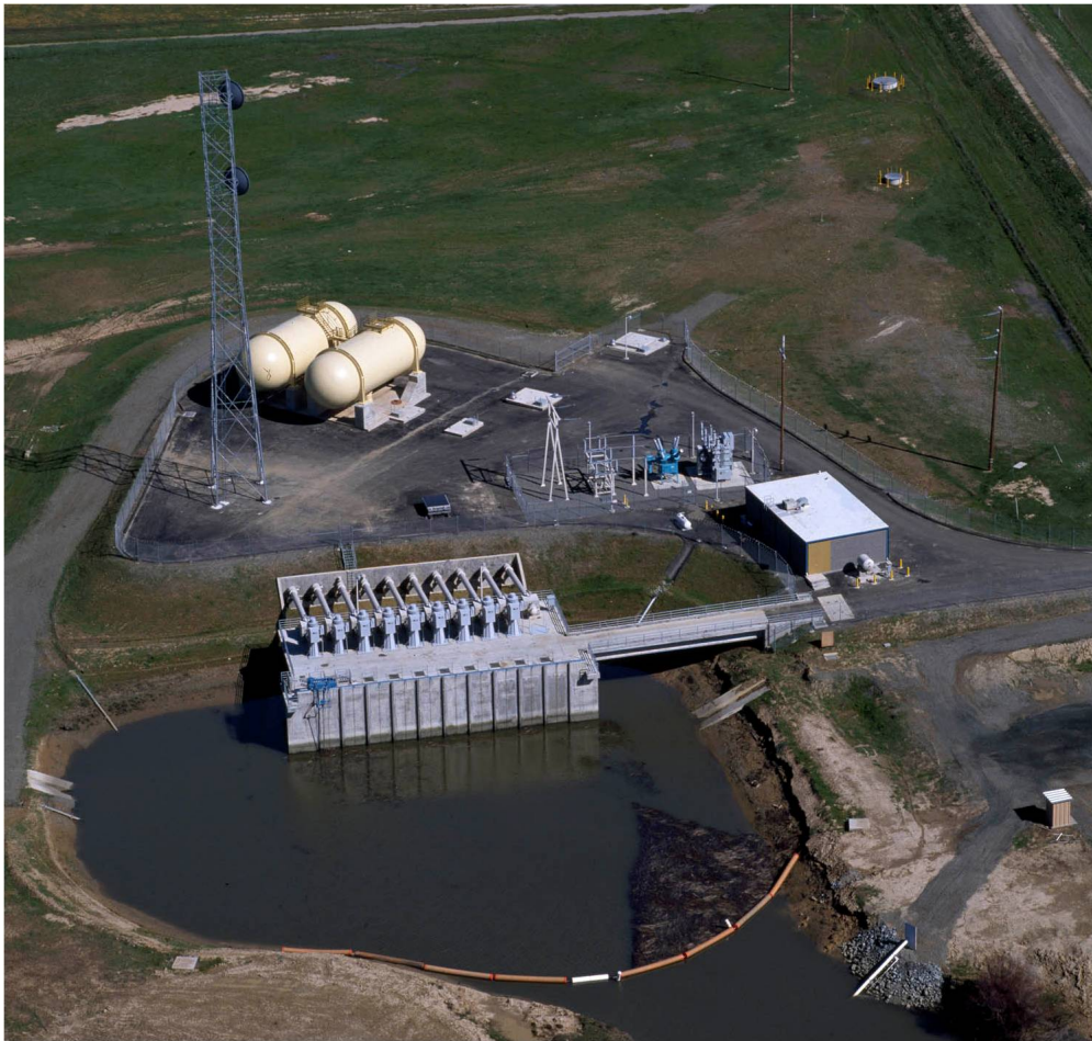
Exhibit 4. Aerial view of Barker Slough Pumping Plant.
