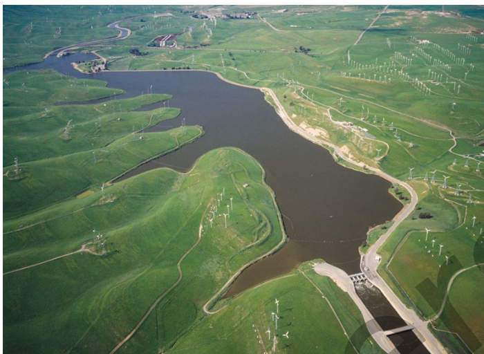
Bethany Reservoir and the start of the California Aqueduct
