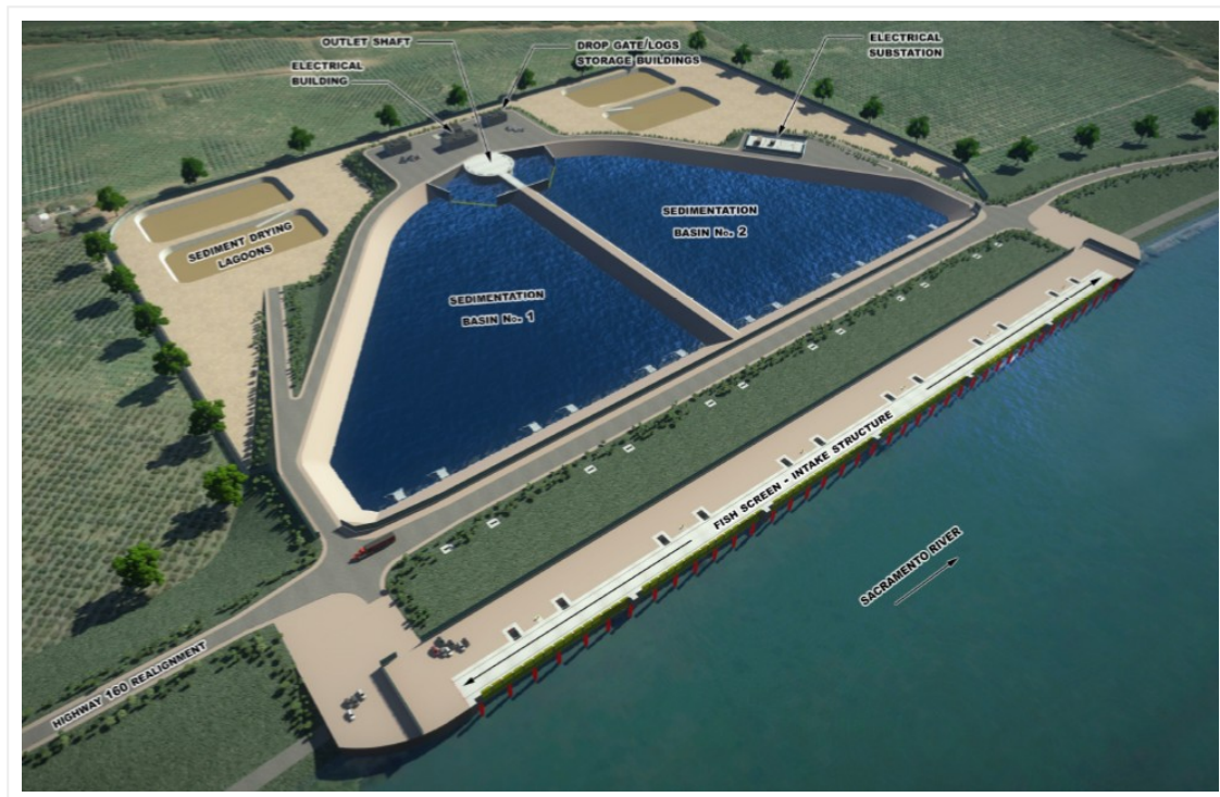
— Figure 1. Conceptual rendering of one of the three on-bank intake facilities on the Sacramento River for the Twin-Tunnels project (Figure 3-19a from the 2016 Final EIR/EIS).
