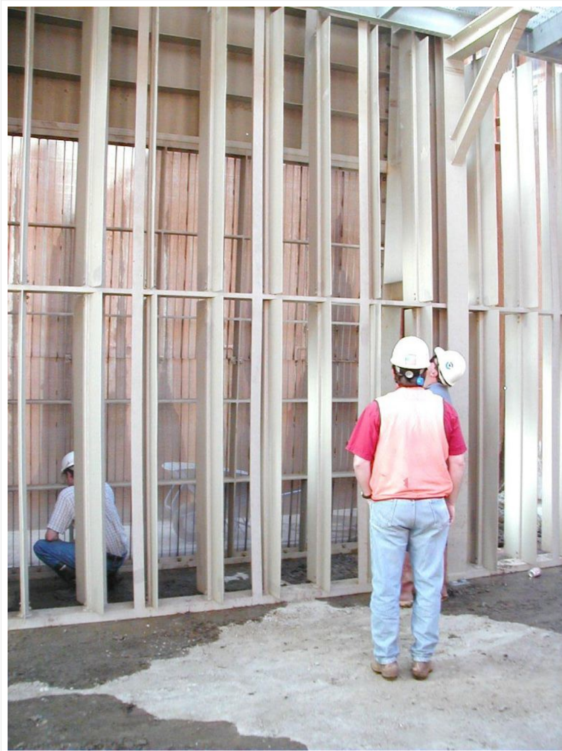
— Figure 1. Picture of flow-control baffles in the open position (foreground) and flat-plate screens in the background. Entire structure dewatered during construction. Picture by Dave Vogel.
