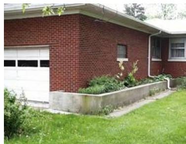
This home has a floodwall to protect it from low level flooding.
