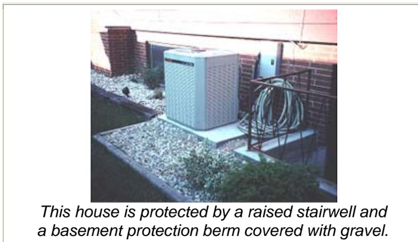
Sump pumps cannot keep up with surface water. If you have sandy or permeable soil, you should consult an engineer or soils expert to ensure that the berm will extend far enough away from the walls. Note: check local permit requirements before filling or grading a yard.
