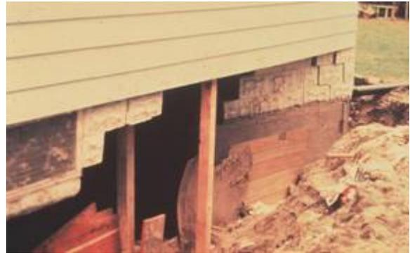
Dry floodproofing is not recommended for keeping surface water out of a basement. The water pressure can break the walls and floor.
