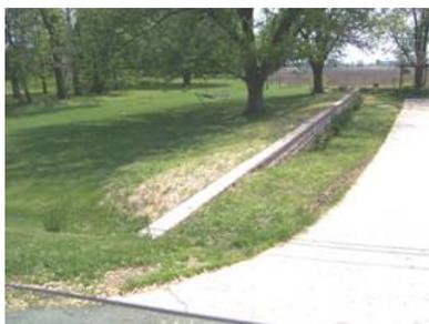
This berm protects the home from flooding from the stream to the left.
