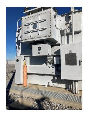
**Photo 23.** Transformer and compressed nitrogen tank in the center subsection of the Marshall Substation.
