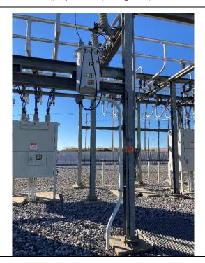
**Photo 13.** Mounted transformer in the center subsection of the Marshall Substation.
