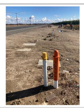
**Photograph 14.** PG&E natural gas pipeline markers along the northern border of the project site (facing east).
