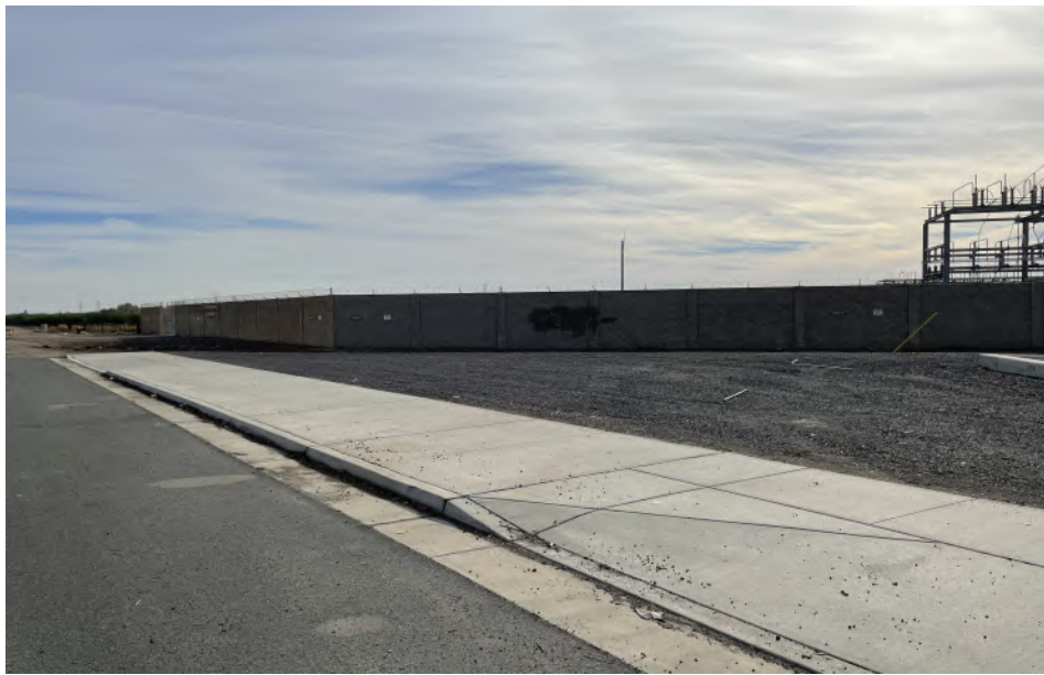
Photo A: View east/southeast from Claribel Road to existing perimeter wall of electrical substation (located 300 feet away)
