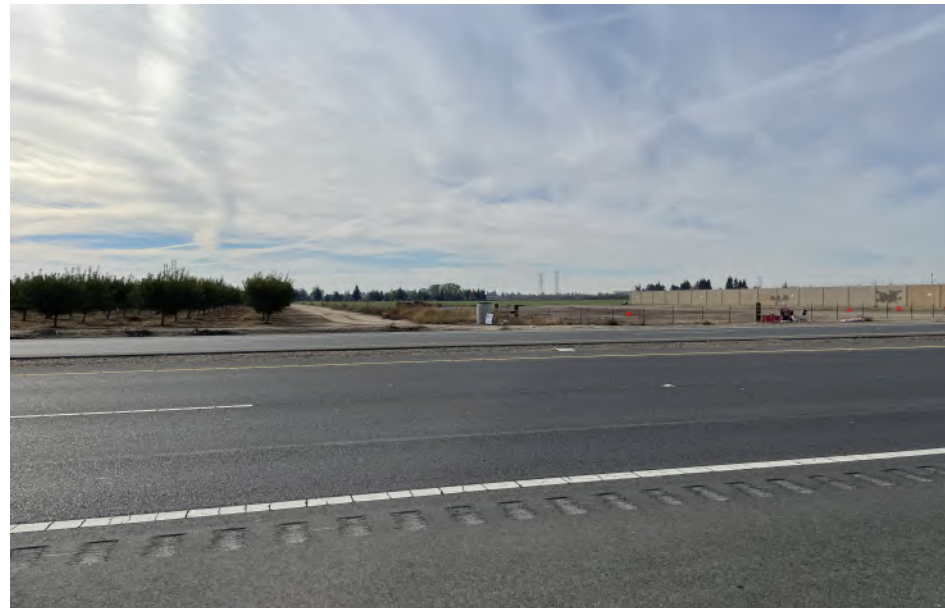
Photo C: View southwest from WB Claribel Road to proposed facility site (located 150 feet away)
