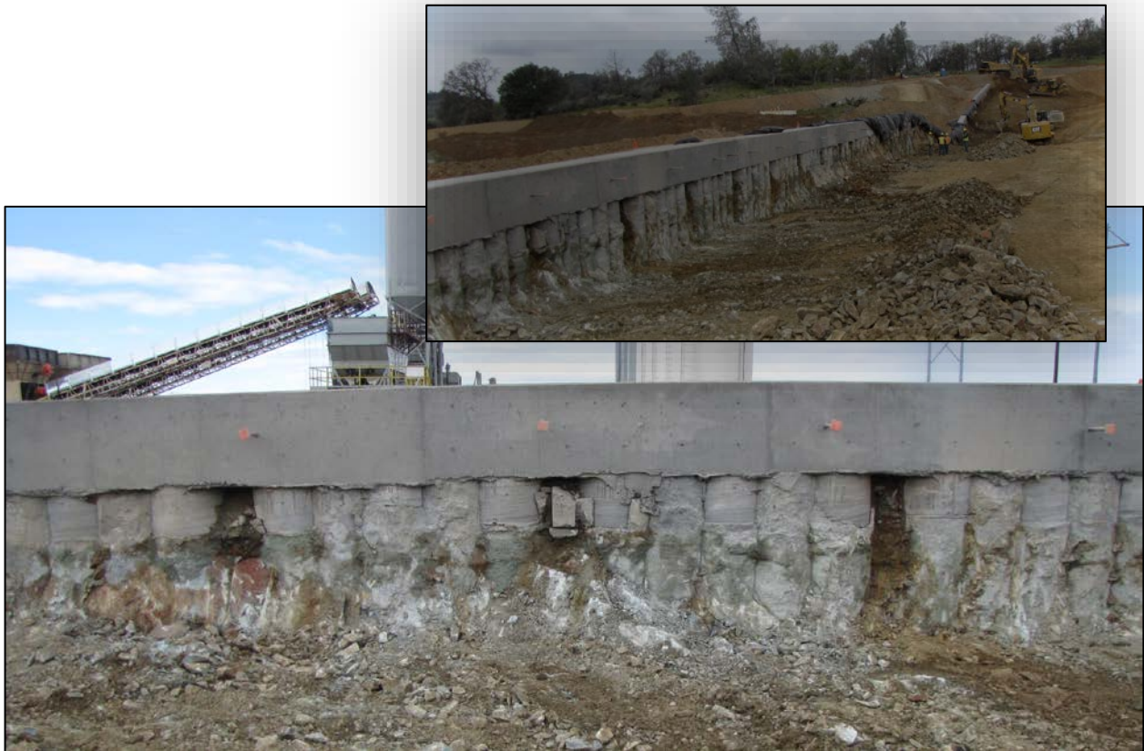
Figure 1. Photographs of Emergency Spillway Control Section (Top) and Secant Pile Wall (Bottom)
