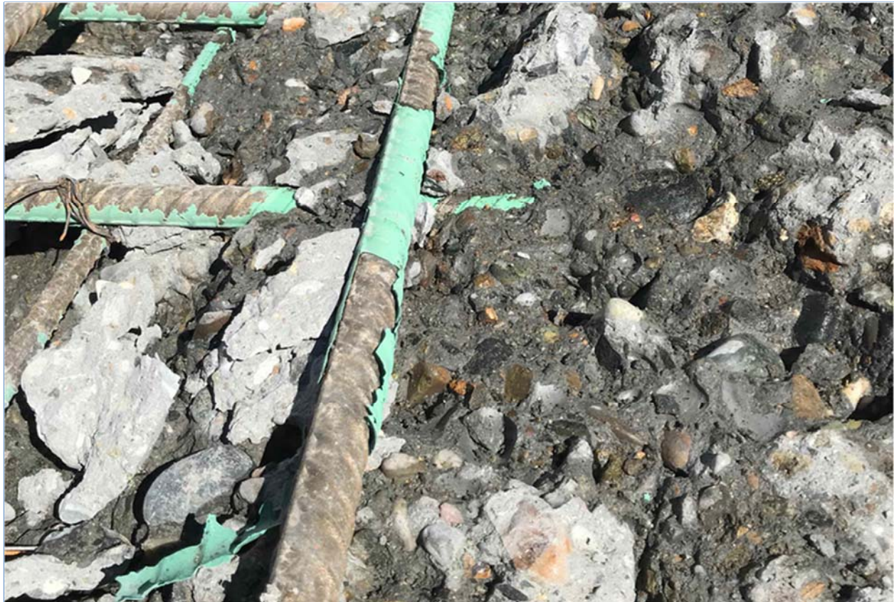
Figure 3. Photographs of the hydro-demolition equipment used on the FCO chute slab (top), and the excavated surface showing exposed aggregate tenaciously bonded to slab.
