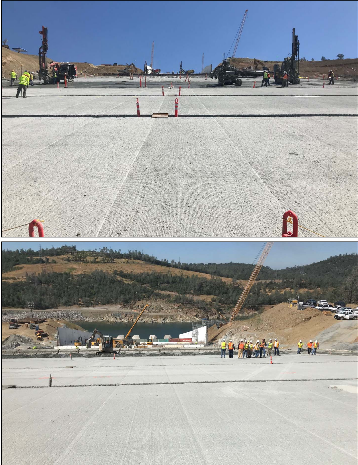
Figure 2. Photos showing RCC spillway walls removed from the FCO and the milled RCC foundation looking upstream (top), and downstream (bottom).
