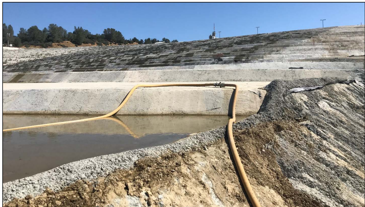
Figure 1. Photographs of the completed demolition work at the upper section of the FCO chute (top) and the RCC apron at the Emergency Spillway (bottom).
