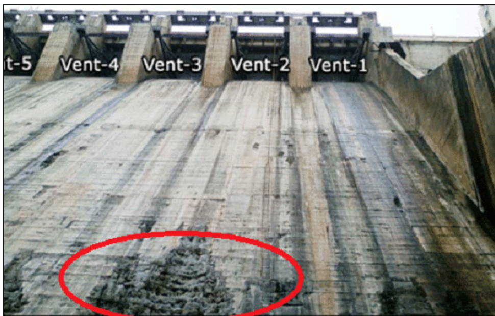
Figure 4. Example of cavitation damage in an open channel spillway chute (Source: The Constructor – “Cavitation Damage to Concrete Structures Prevention Methods”)
