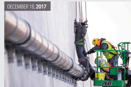
Drainage system. Drainage pipes are connected to the outer sidewalls of the upper chute of the main spillway.
