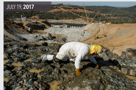
Cleaning bedrock. Workers remove loose rocks and debris in preparation for placement of concrete on the upper chute of the main spillway.
