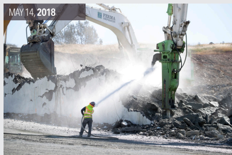
Middle chute berm demolition. Temporary RCC sidewalls are removed from main spillway prior to placement of permanent structural concrete walls.
