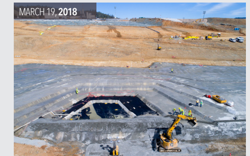
Construction of RCC splashpad. Armored the hillside between the emergency spillway and secant pile wall to prevent erosion should the emergency spillway flow.
