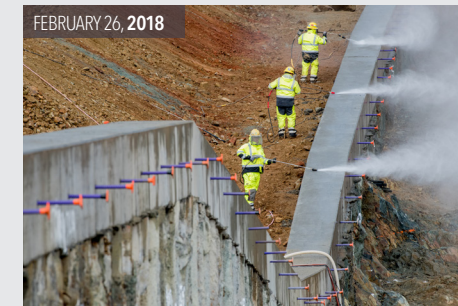
1,450-foot secant wall. A concrete beam anchored to the top of the secant pile wall forms the base of the roller-compacted concrete splashpad.
