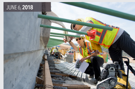
Inspection work. DWR engineers check the leading edge of the upper chute where new structural concrete work will be poured on main spillway.
