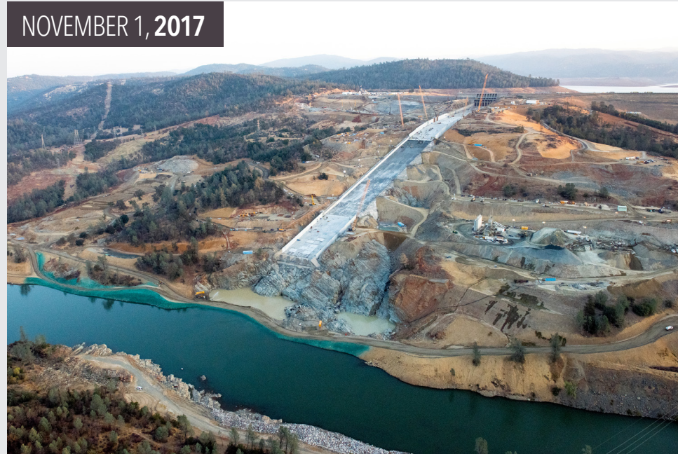
Phase 1 repairs to main spillway allowed outflows of 100,000 (cfs), if necessary, during upcoming winter season.
