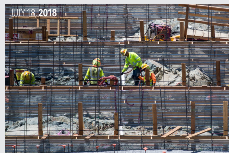
Stay-forms. Workers prepare for placement of leveling concrete on the upper chute of the main spillway.
