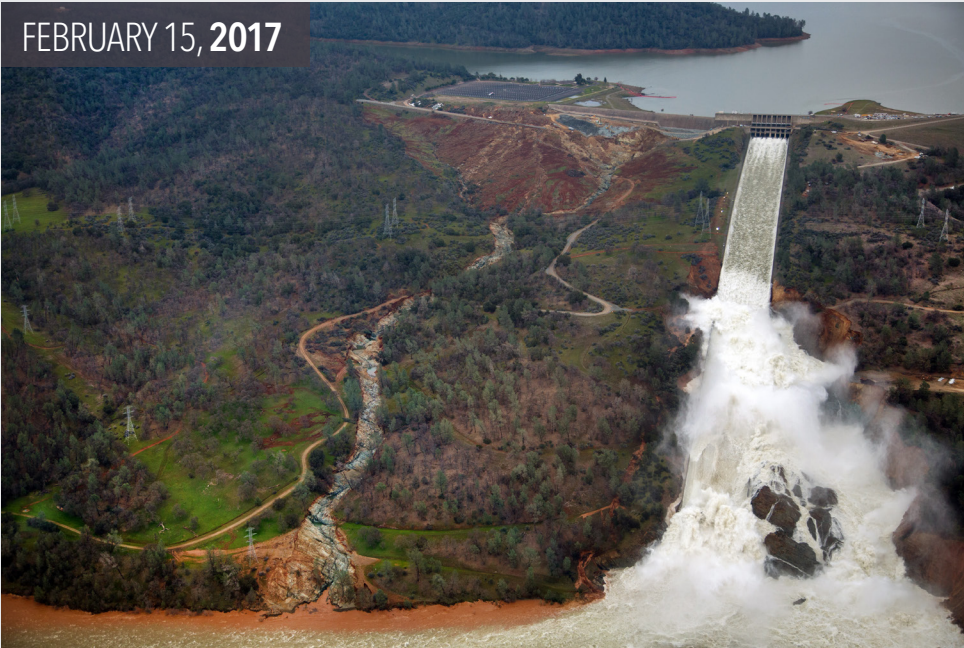
Lake Oroville damaged main spillway with an outflow of 100,000 (cfs).
