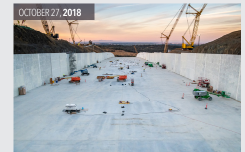
Concrete finishing. Workers dry finish concrete slabs and sidewalls on the upper chute of the main spillway.
