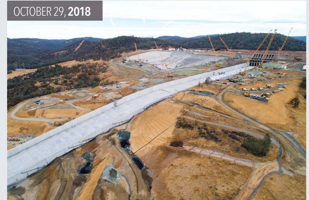
Final concrete work on the upper chute of main spillway and the emergency spillway.
