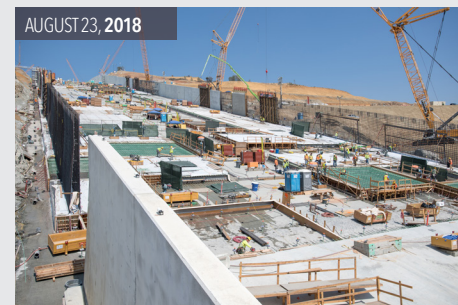
Structural concrete. Crews place structural concrete on middle and upper chutes of the main spillway.
