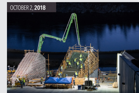
Energy dissipator repair. Concrete is placed atop an energy dissipator block on the lower chute of the main spillway.
