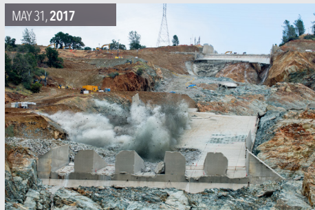
Controlled blasting. A detonation breaks up concrete from the lower chute of the damaged main spillway.
