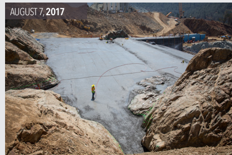
Roller-Compacted Concrete (RCC). To facilitate curing, water is sprayed on RCC in an erosion area between the upper and lower chutes of the main spillway.
