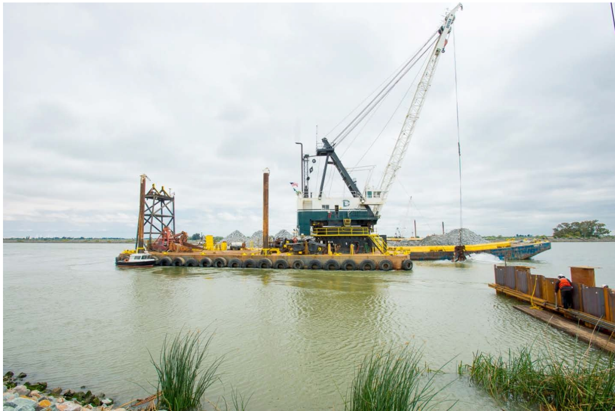
Figure 3-4 Rock Placement During EDB Installation
