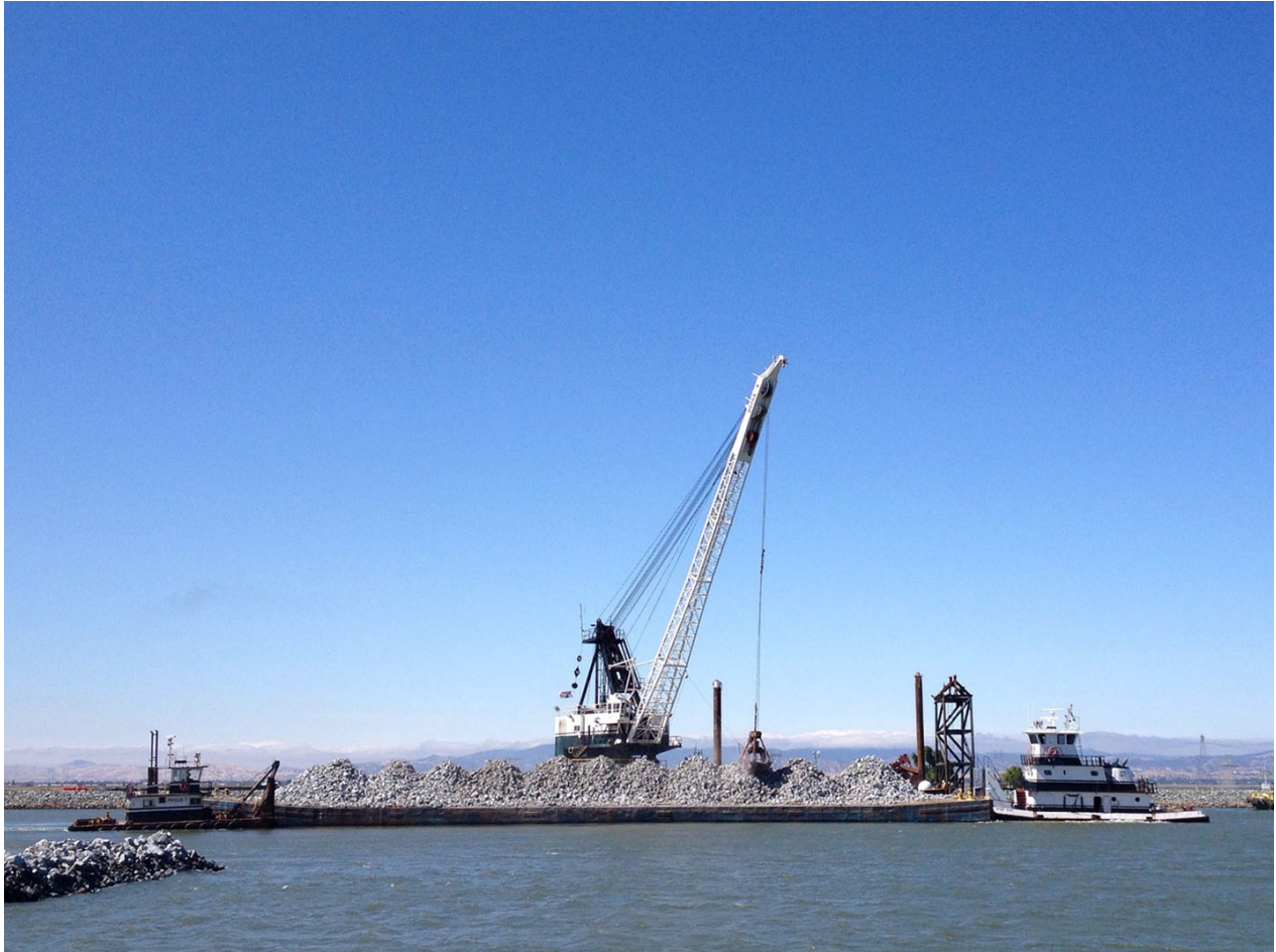
Figure 3-5 Rock Placement During EDB Installation
