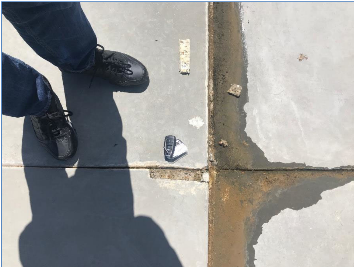
Figure 4. Photographs Taken During BOC Inspection of FCO
