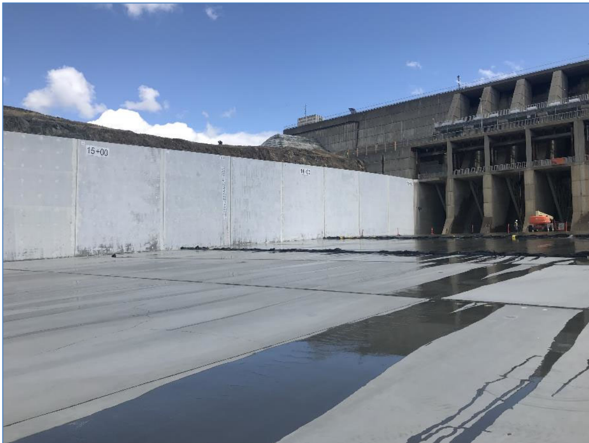
Figure 1. Photographs Taken During BOC Inspection of FCO
