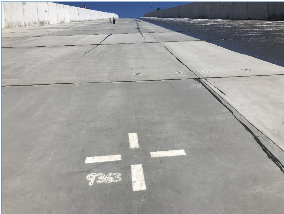
Figure 3. Photographs Taken During BOC Inspection of FCO
