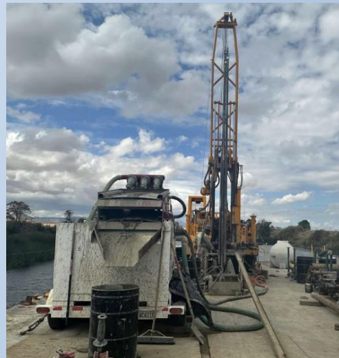
Photo from October 2025 overwater geotechnical investigations
