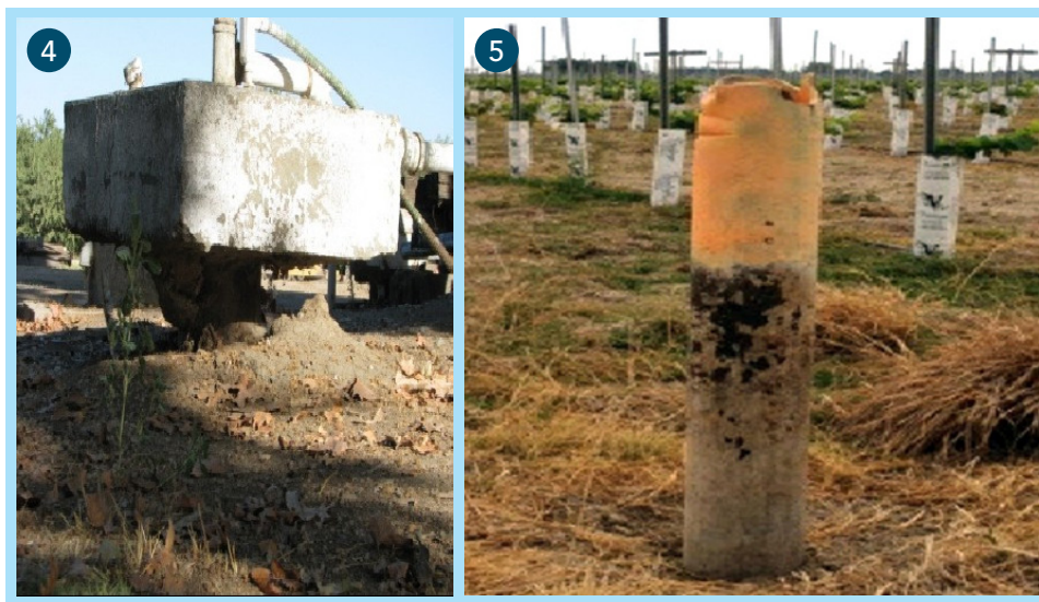
Figures 4 and 5. Subsidence near El Nido has exposed the underside of a concrete pad supporting a water well (left) and the casing of an abandoned gas well (right) (LSCE et al., 2014).
