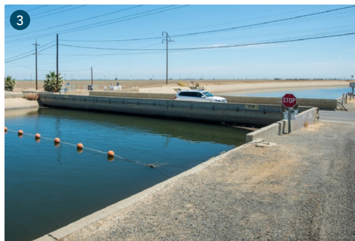
Figure 3. Subsidence near Firebaugh in Fresno County has lowered the surrounding land, causing water levels in the Delta-Mendota Canal to reach the underside of a bridge crossing the canal, illustrating the impact of subsidence on infrastructure.
