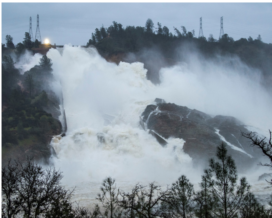
The California Department of Water Resources continues an outflow of 80,000 cubic feet per second from the damaged Lake Oroville flood control spillway on Friday morning. Photo: DWR, February 17, 2017
