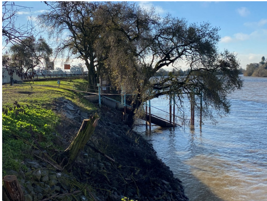
Photo 4. Support piles and 36-inch corrugated metal pipe discharge pipe to be removed on the waterside. Looking south from the levee crown. December 16, 2021
