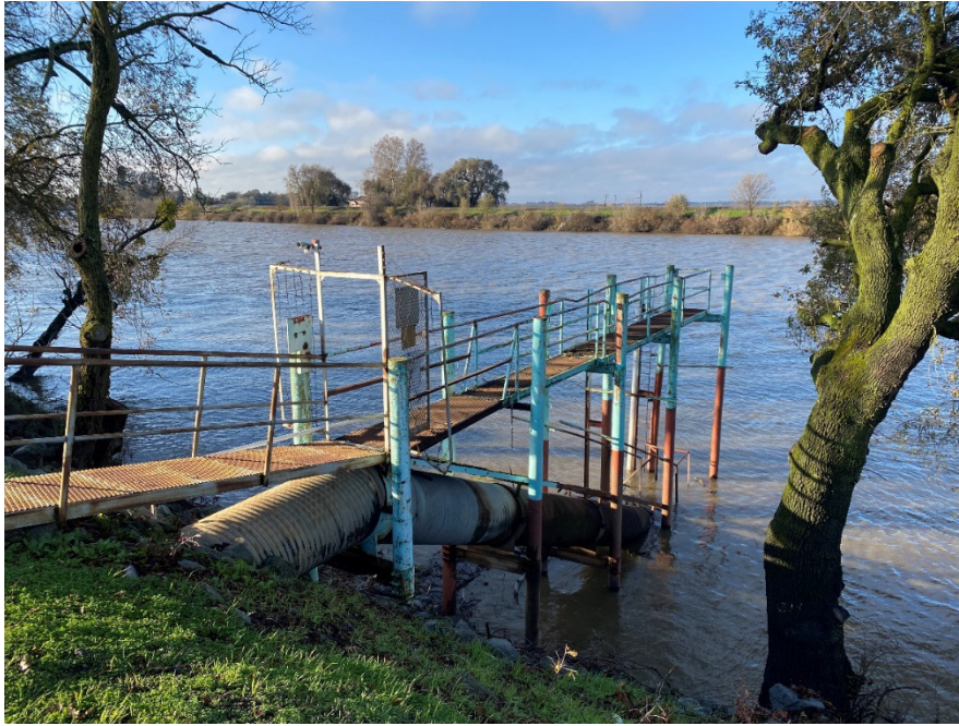
Photo 4. Support piles and 36-inch corrugated metal pipe discharge pipe to be removed on the waterside. Looking south from the levee crown. December 16, 2021
