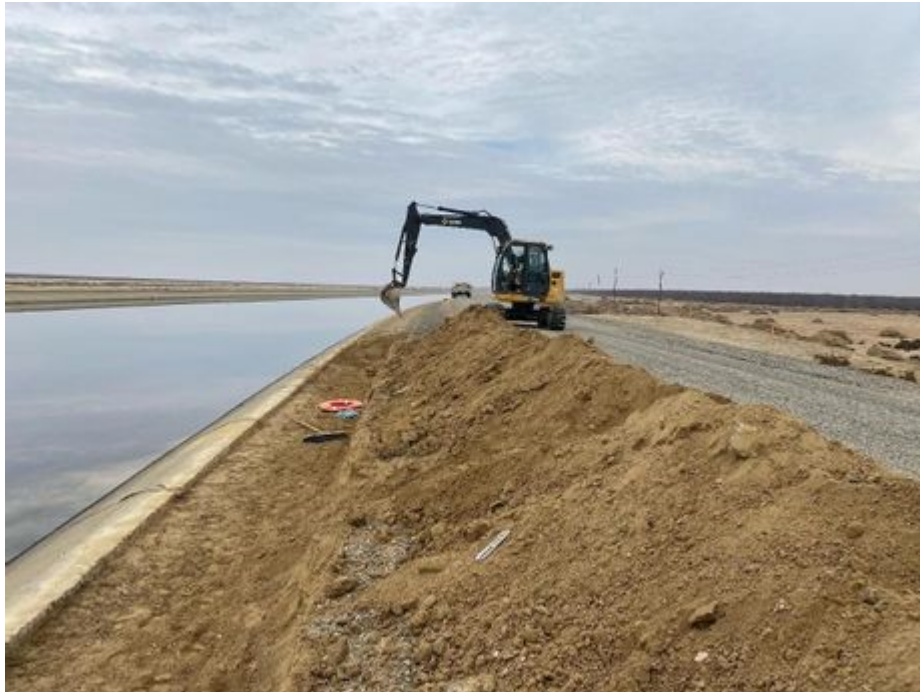
Photo from the Pools 24 and 25 Liner Raise Project
