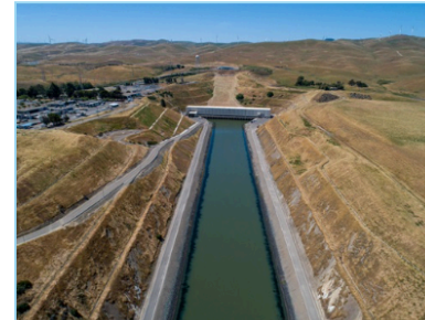
A drone provides a view of the Harvey O. Banks Delta Pumping Plant, the first major plant designed and constructed within the California State Water Project.
