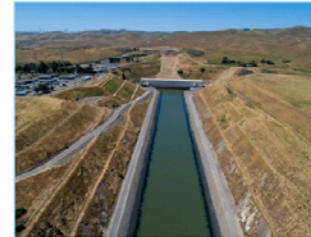
A drone provides a view of the Harvey O. Banks Delta Pumping Plant, the first major plant designed and constructed within the California State Water Project.
