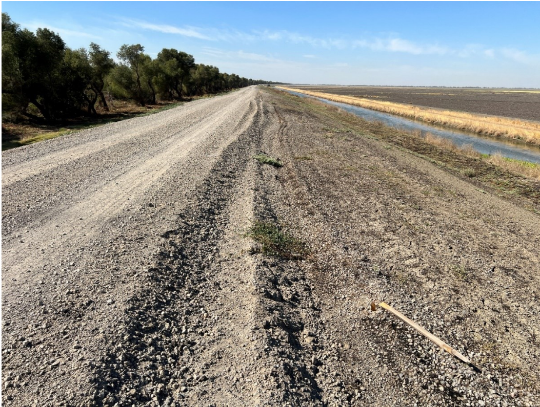
Photo 1. Levee crown - approximate width of 15 feet at LM 15.46.
