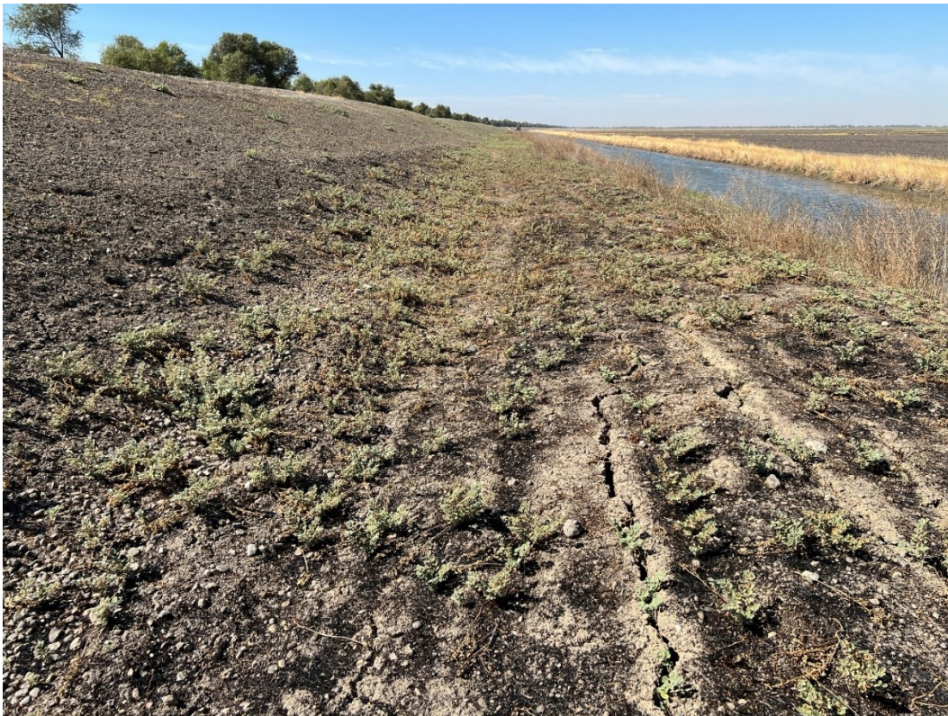
Photo 3. Longitudinal cracking located on landside toe stability berm at LM 15.47.
