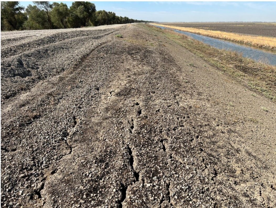
Photo 2. Longitudinal cracking observed on landside slope at LM 15.47.
