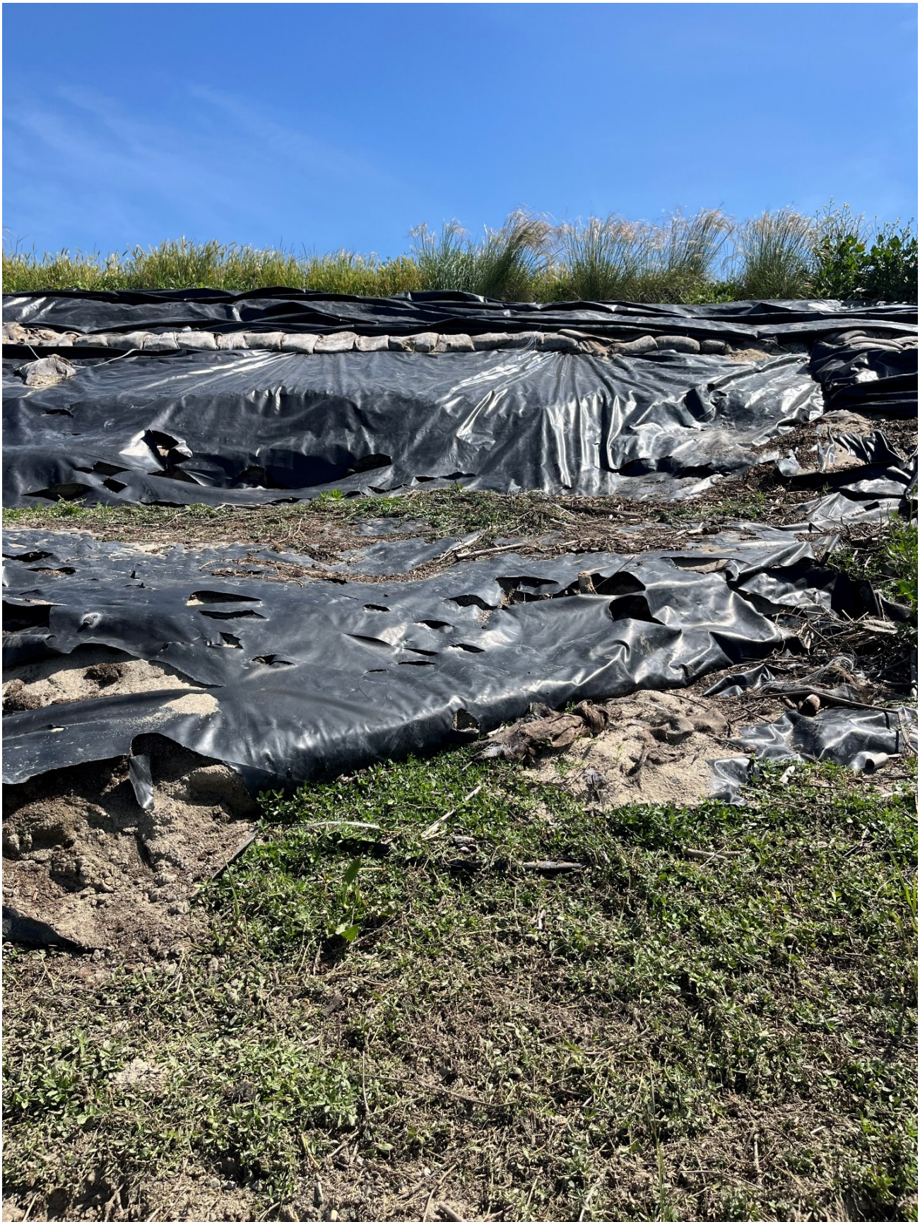
Photo 3: Vertical scarps totaling 6 to 7 feet in height.
