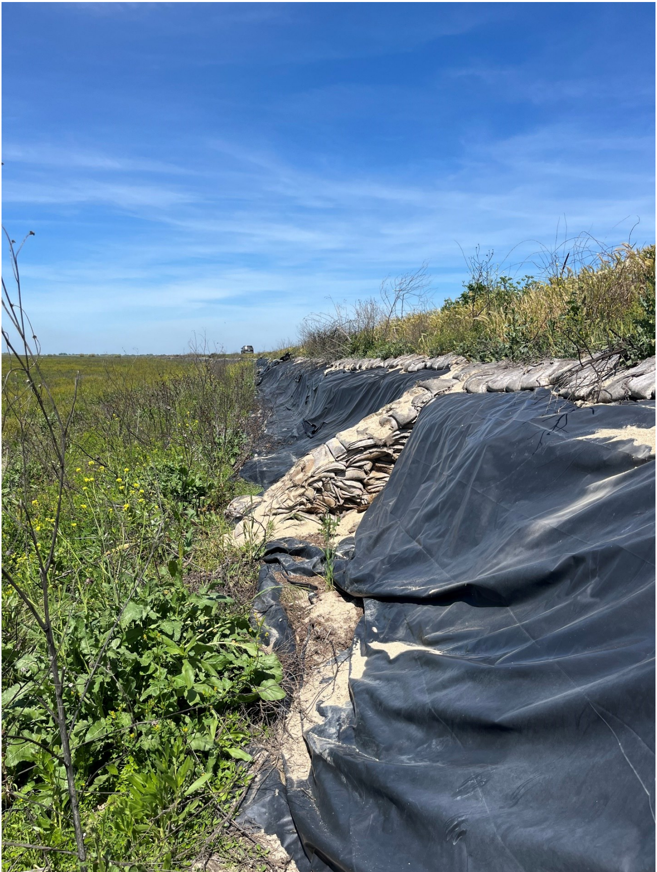
Photo 2: Typical condition, continuous 4-foot vertical scarps.
