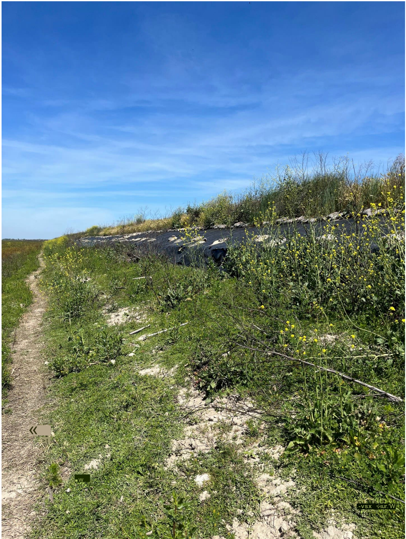
Photo 1: Typical condition, continuous 3-foot vertical scarps.
