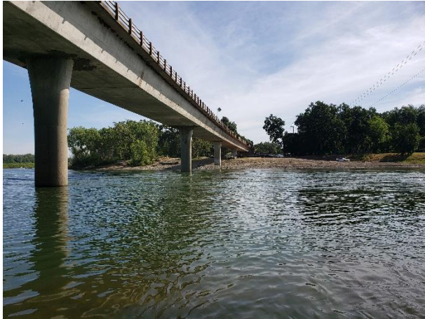
Sacramento River at Woodson Bridge
