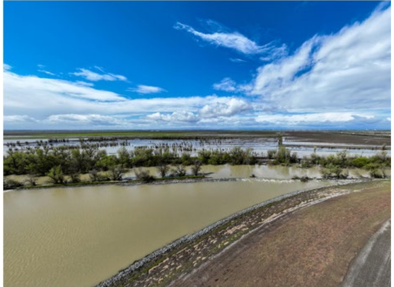
Lower Elkhorn Basin Levee Setback Project
