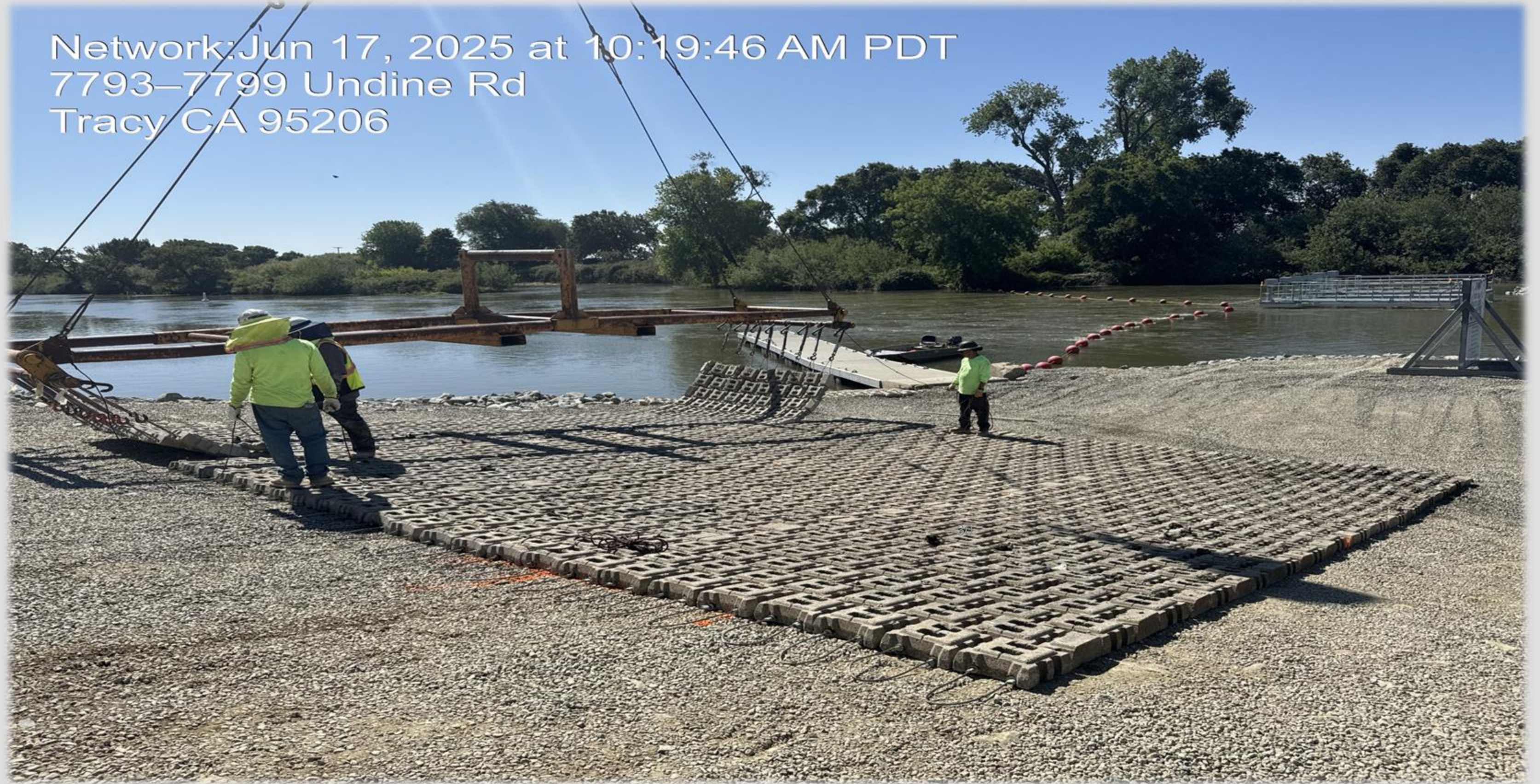
25-01 Temporary Rock Barriers – 2025, 2026, 2027, Middle River, Old River and Grant Line Canal
