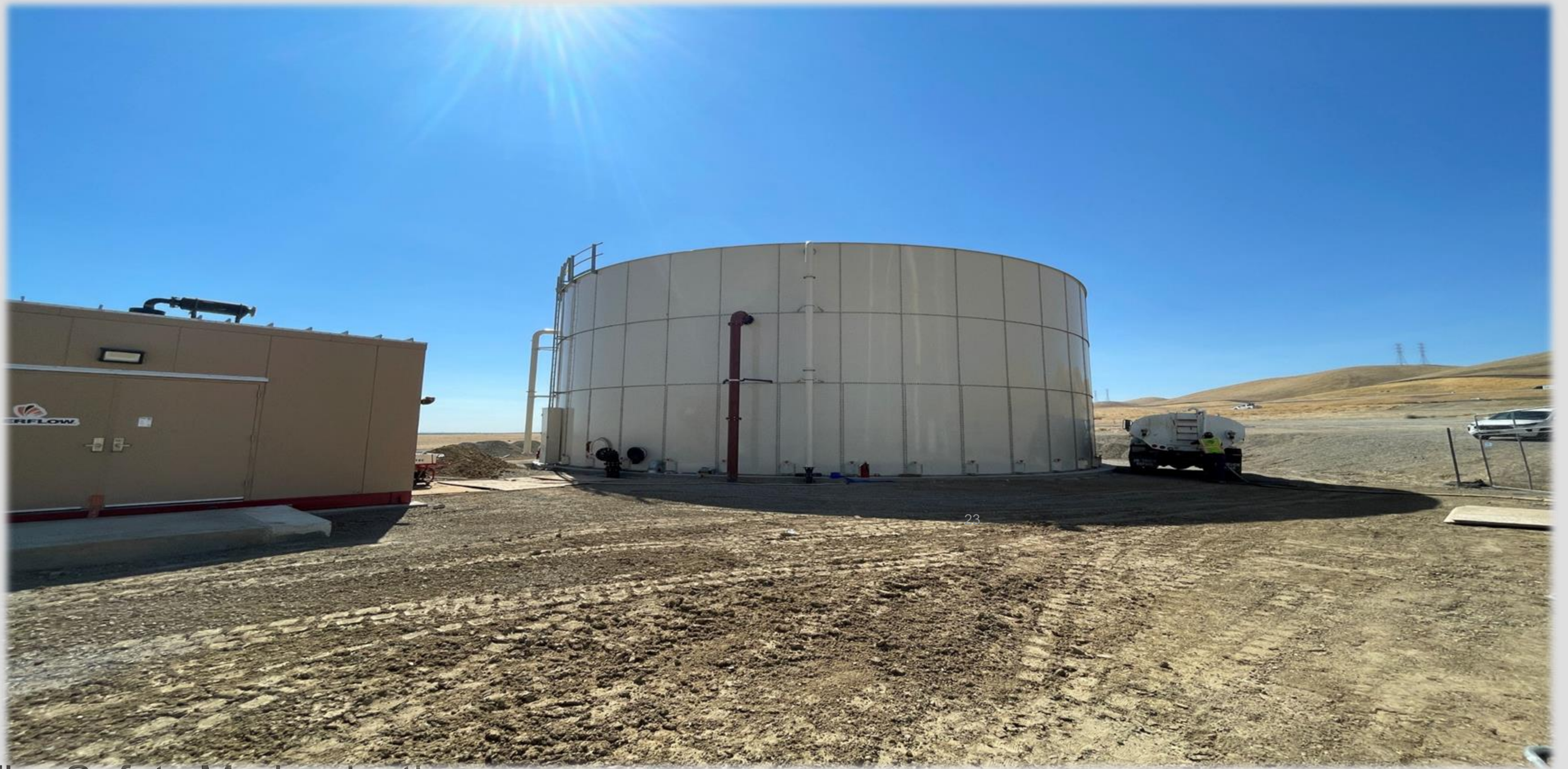
Fire Safety Modernization, Gianelli P/G Plant, SLFD O&M Center, Dos Amigos PP, and Coalinga O&M Center
