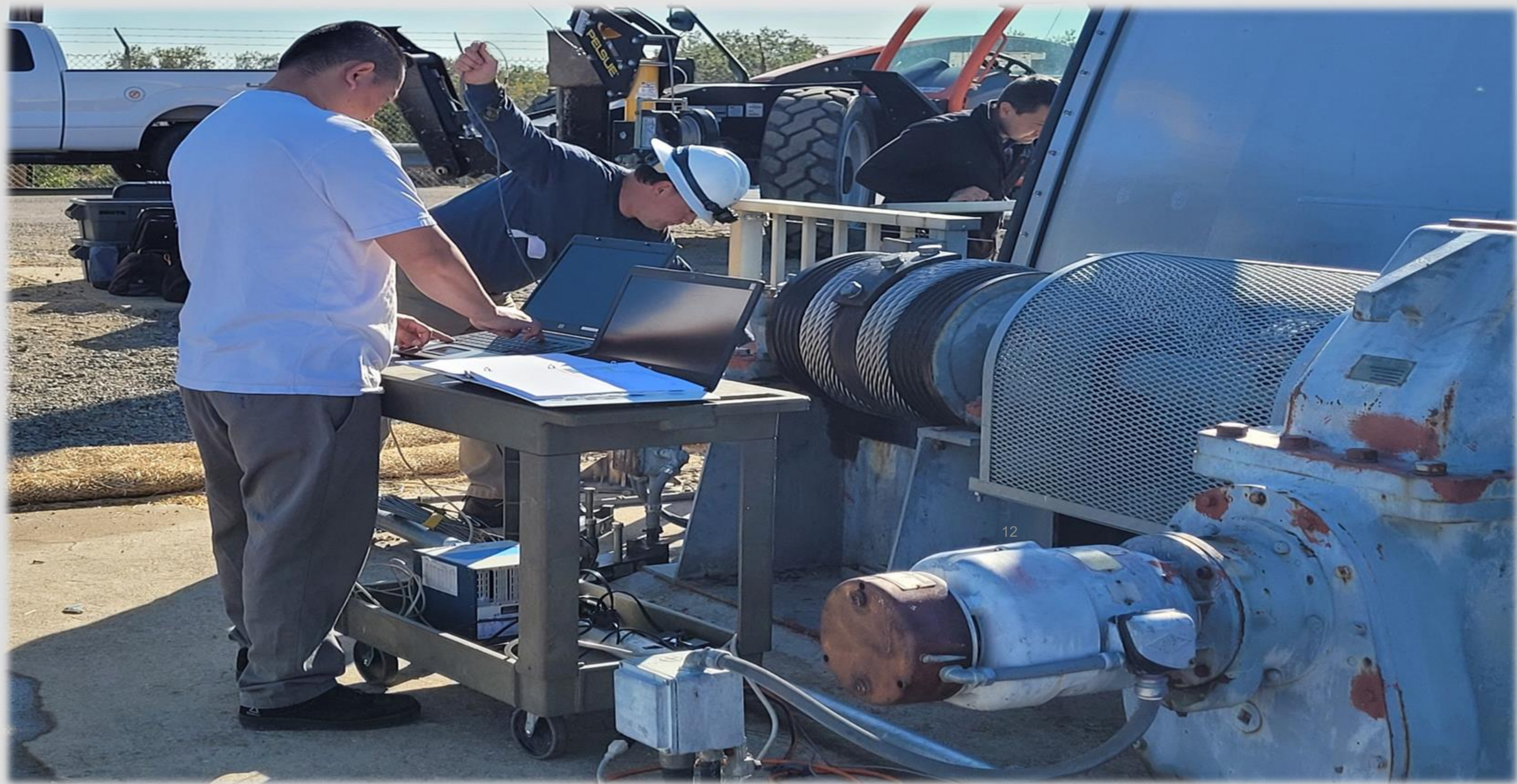
Replacement of Radial Gates, Check Structures 3, 4, 6, and 9
