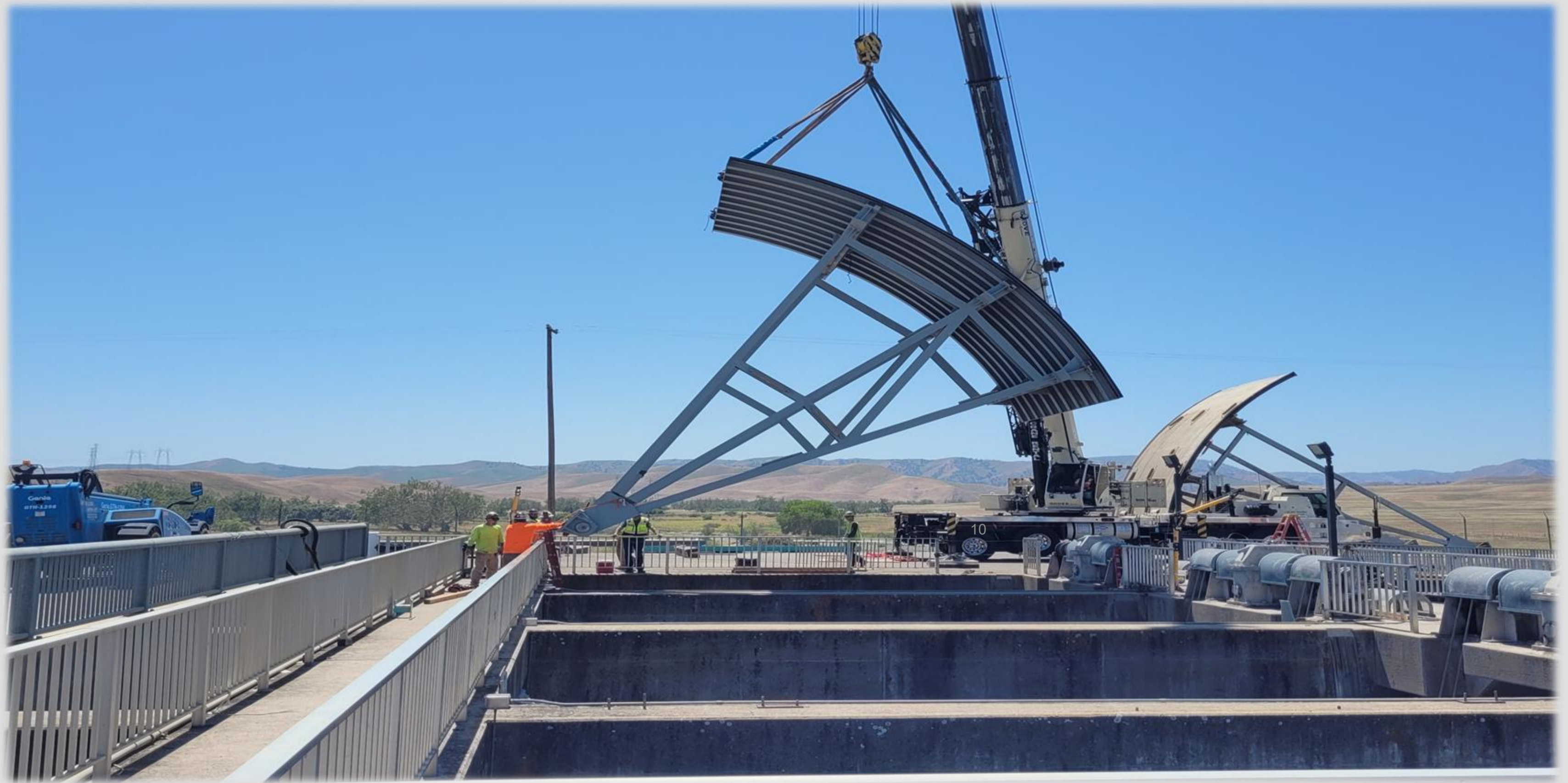
Replacement of Radial Gates, Check Structures 3, 4, 6, and 9
