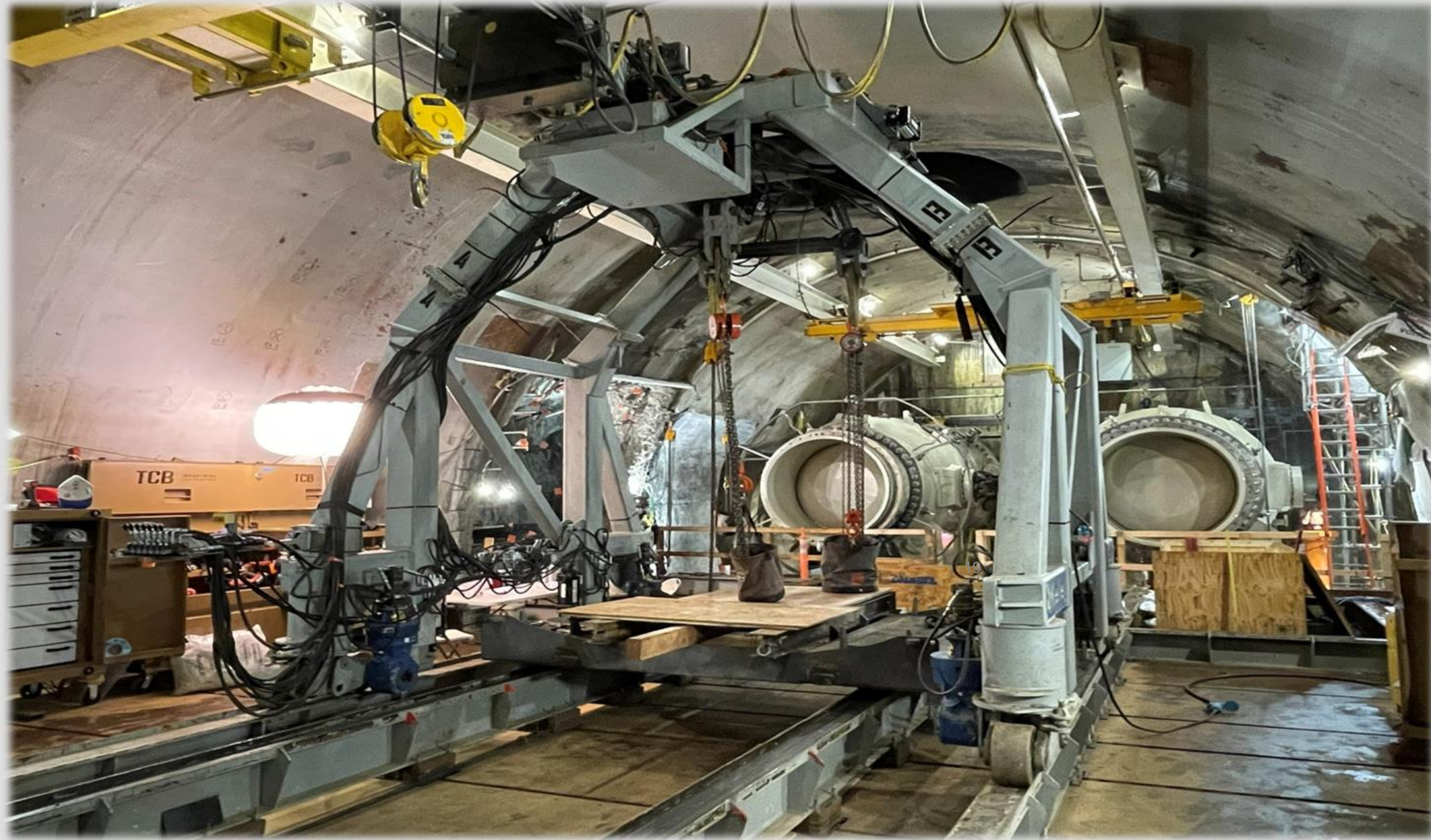
River Valve Outlet System Rehabilitation, Oroville Dam Diversion Tunnel No. 2
