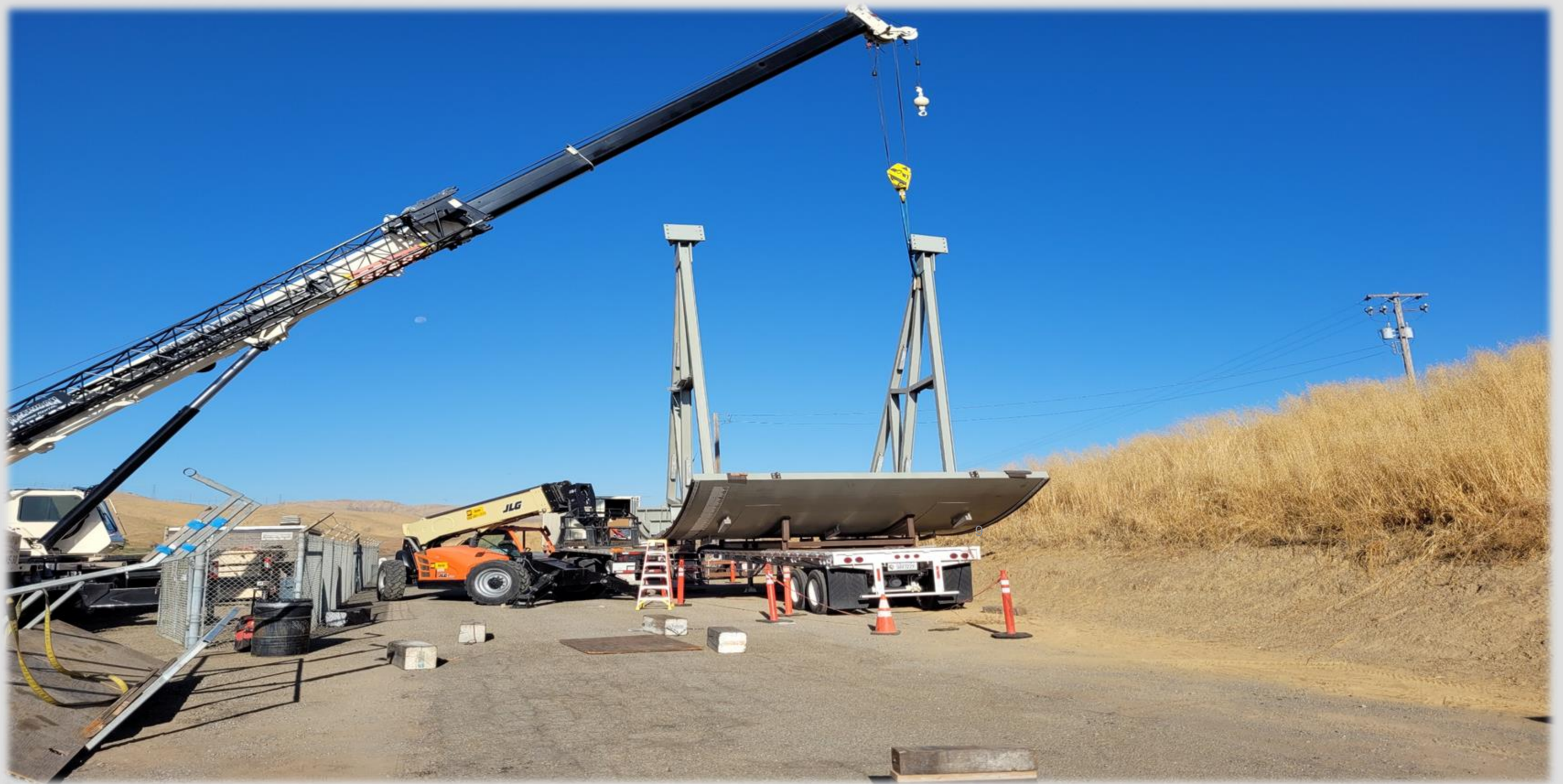
Replacement of Radial Gates, Check Structures 3, 4, 6, and 9
