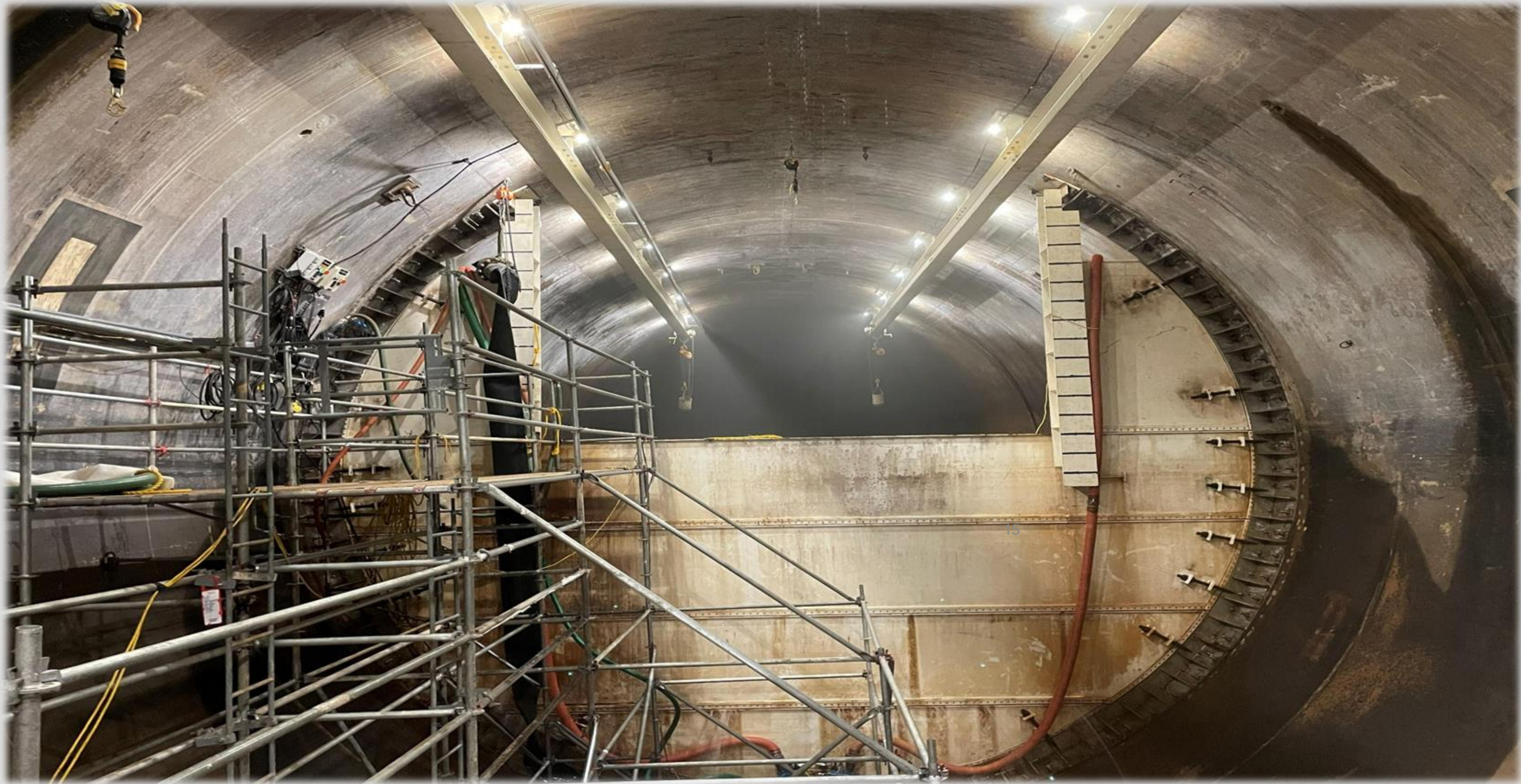
River Valve Outlet System Rehabilitation, Oroville Dam Diversion Tunnel No. 2
