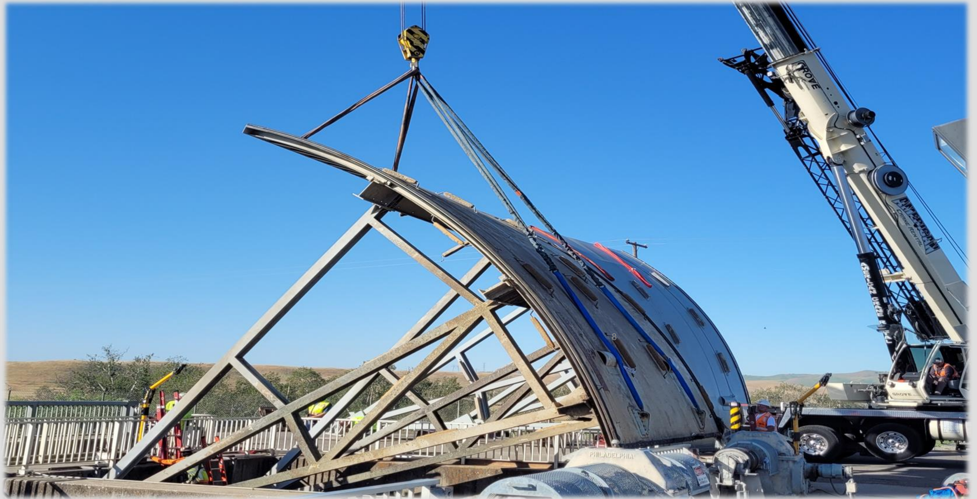
Replacement of Radial Gates, Check Structures 3, 4, 6, and 9
