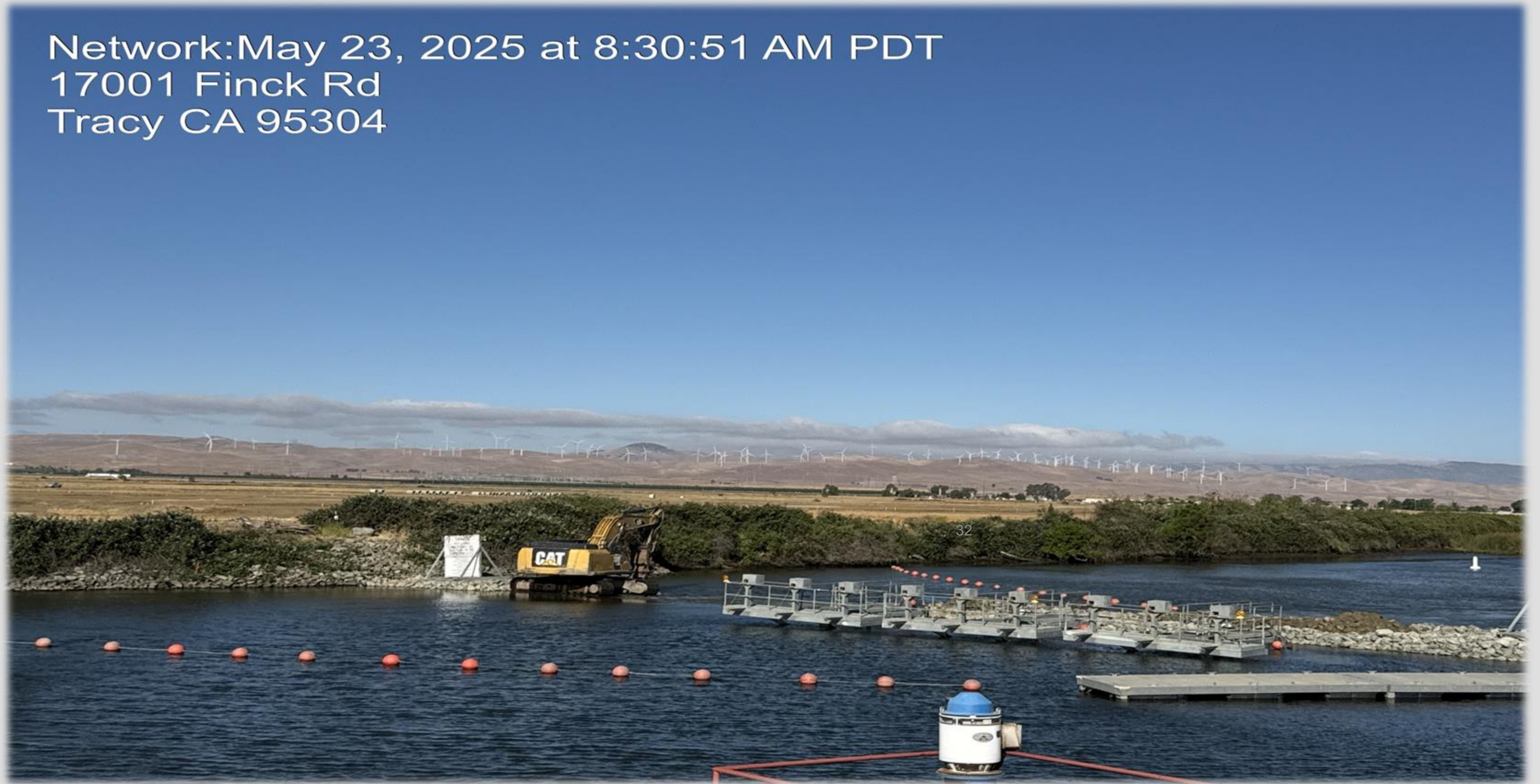
25-01 Temporary Rock Barriers – 2025, 2026, 2027, Middle River, Old River and Grant Line Canal
