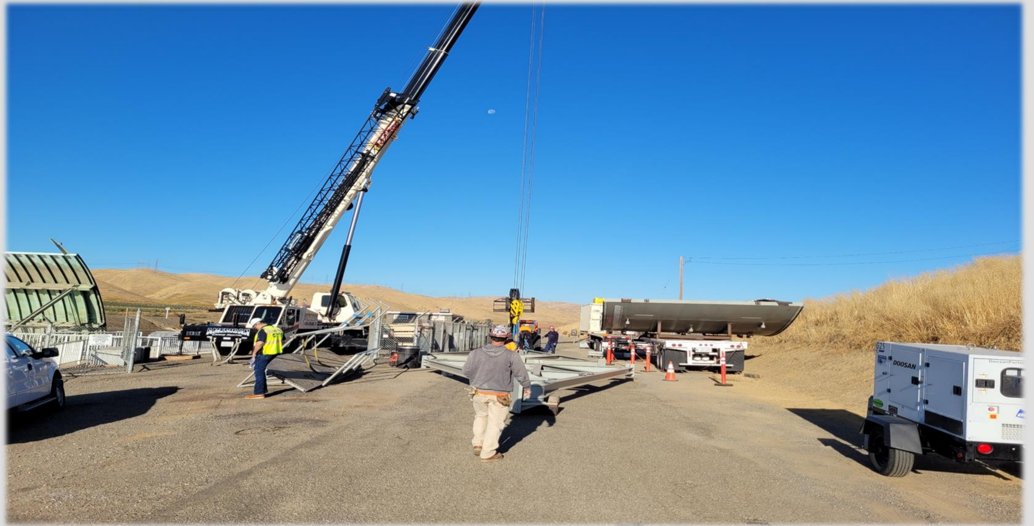
Replacement of Radial Gates, Check Structures 3, 4, 6, and 9
