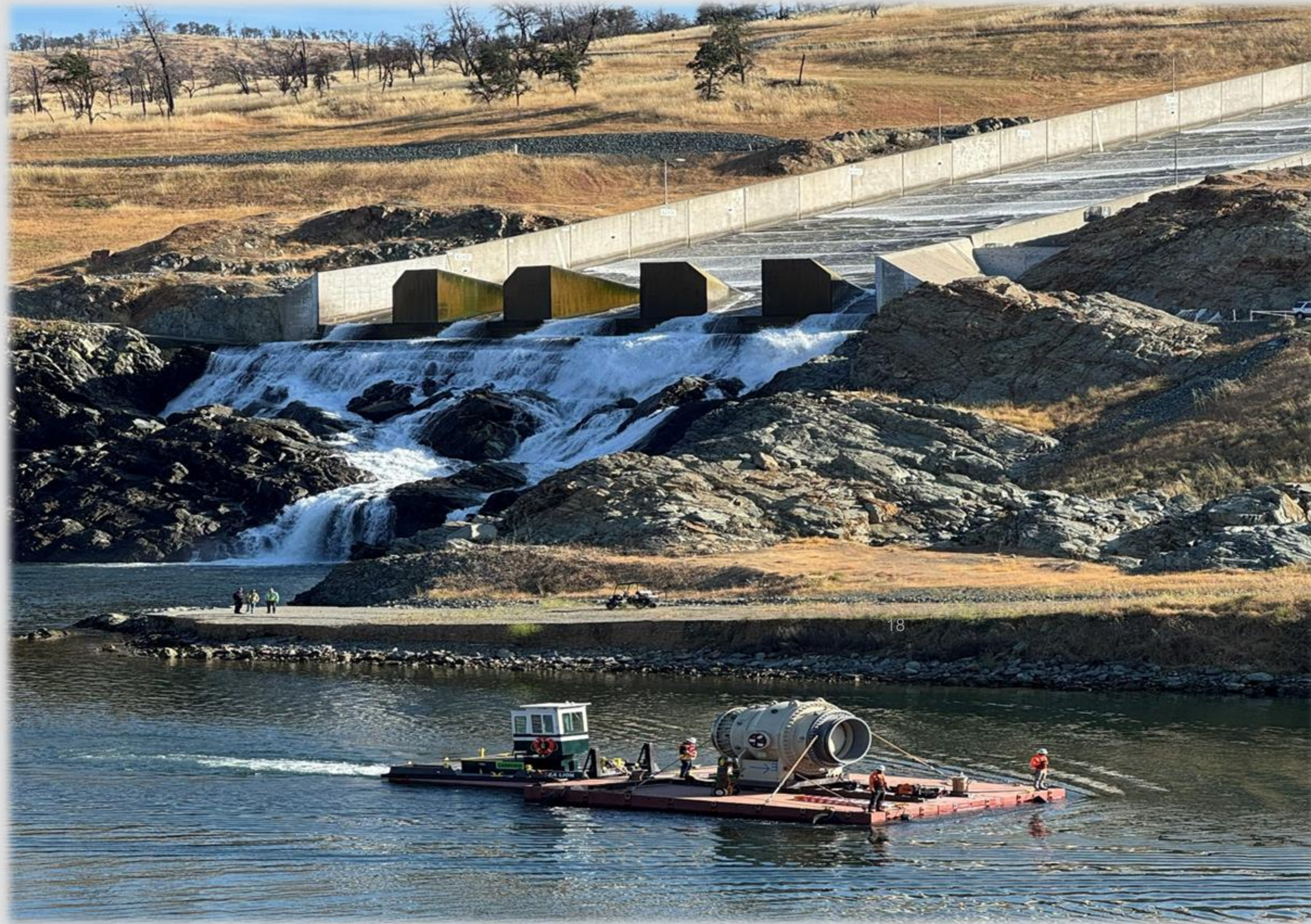
River Valve Outlet System Rehabilitation, Oroville Dam Diversion Tunnel No. 2
