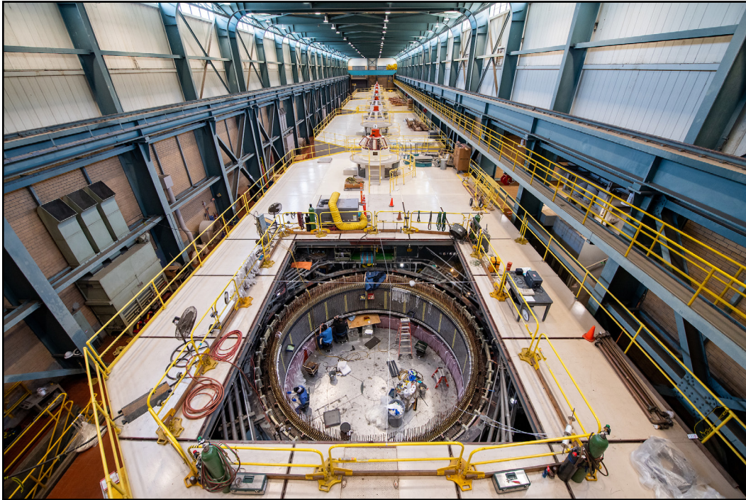
An inside view during motor refurbishment work for one of the units in William R. Gianelli Pumping-Generating Plant which pumps water from O'Neill Forebay into the San Luis Reservoir. Water is released through the plant in generating mode when service area demands are in excess of direct Delta diversions. The San Luis Complex is a joint-use facility between U.S. Bureau of Reclamation and California Department of Water Resources. Photo by Kelly M. Grow/DWR.
