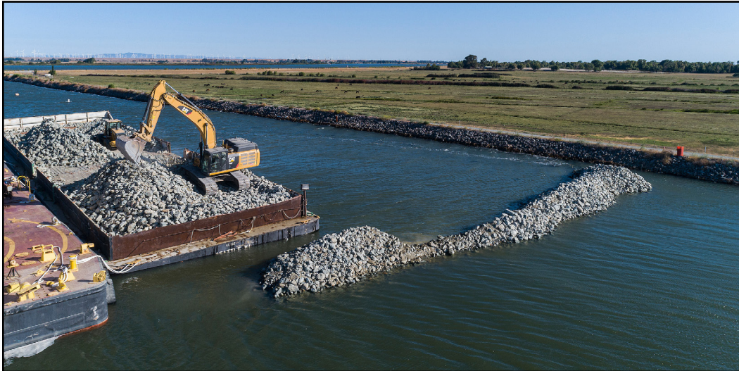
Construction crews working on the temporary emergency drought barrier for the West False River in the Sacramento-San Joaquin Delta in Contra Costa County. The 750-foot-wide rock barrier will help deter the tidal push of saltwater from San Francisco Bay into the central Delta. Photo by Andrew Innerarity/DWR.
