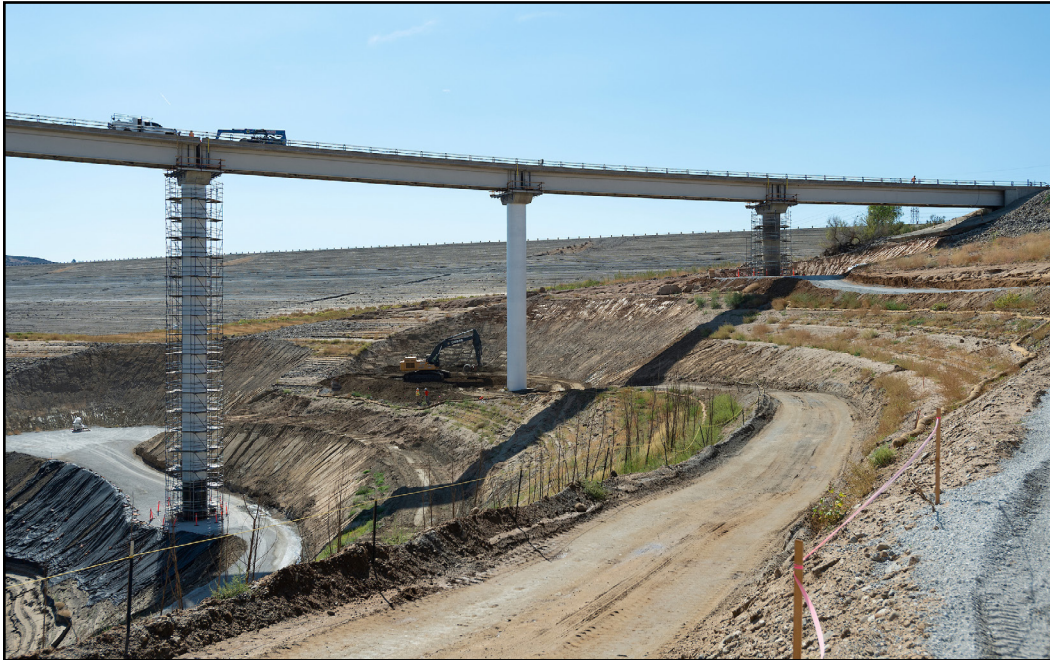
Scaffolding surrounds a partially completed column during this portion of a Castaic Dam Modernization Project whose goal is to allow the facility to better withstand earthquakes' effects by, among other things, wrapping piers with sections of Fiber Reinforced Polymer for the first time. The column in white is a completely wrapped section. Photo by Andrew Innerarity/DWR.
