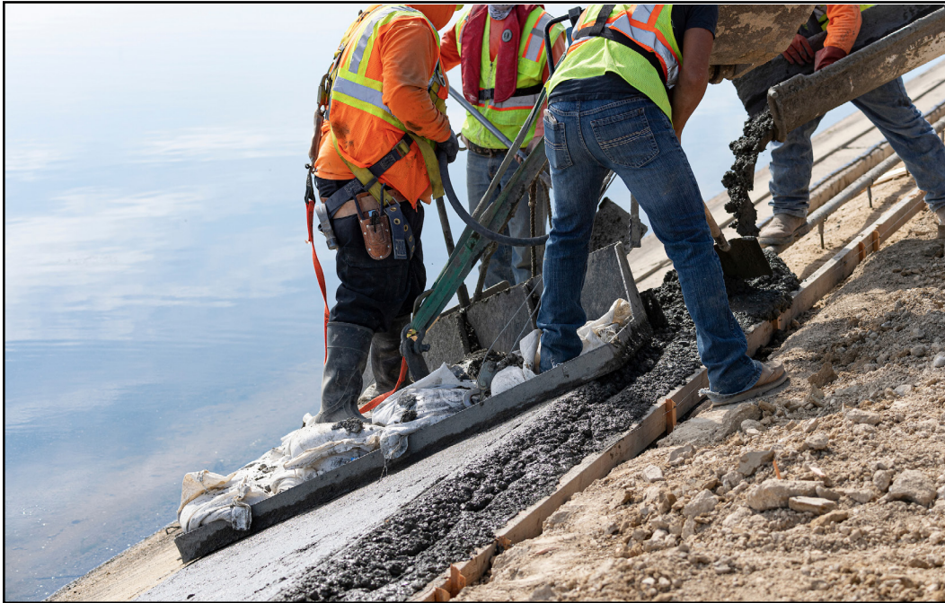
In this photo from March 9, 2021, Bosco Constructors personnel lay concrete as subsidence repair work takes place on the California Aqueduct near Lost Hills in Kern County. Photo by Andrew Innerarity/DWR.
