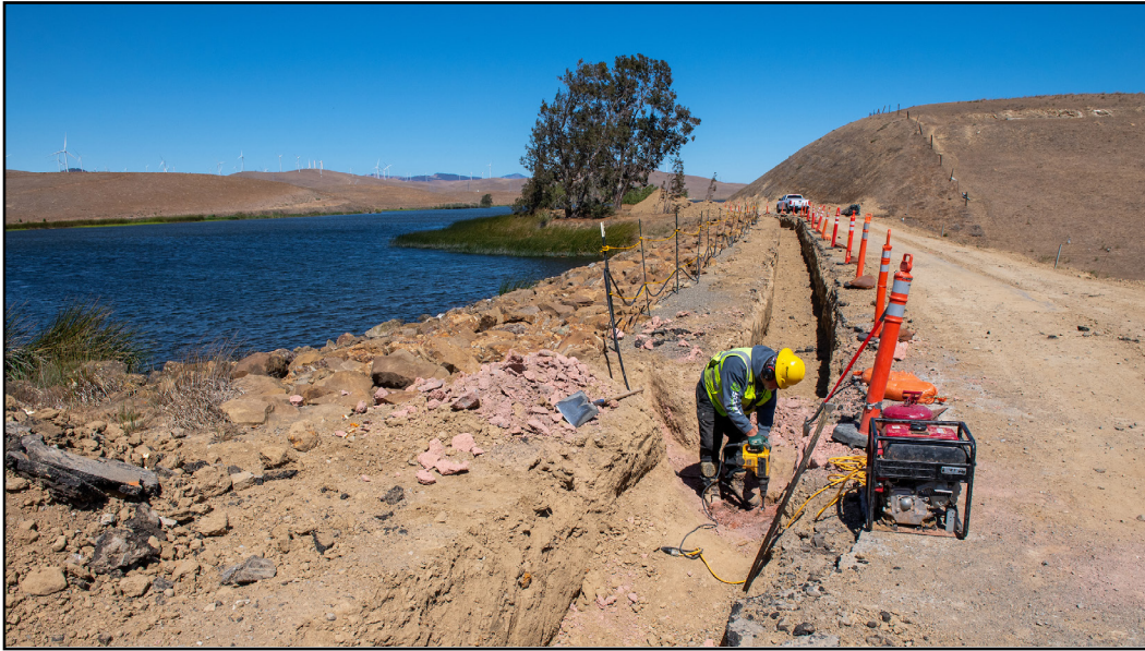
The Department of Water Resources, along with independent contractors, continue work on restoration measures at Bethany Reservoir. These measures include excavating and backfilling each downstream dam face to repair rodent holes and erosion areas. Bethany Reservoir is part of the State Water Project and is located 10 miles northwest of Tracy, Calif. Photo by Kelly M. Grow/DWR.
