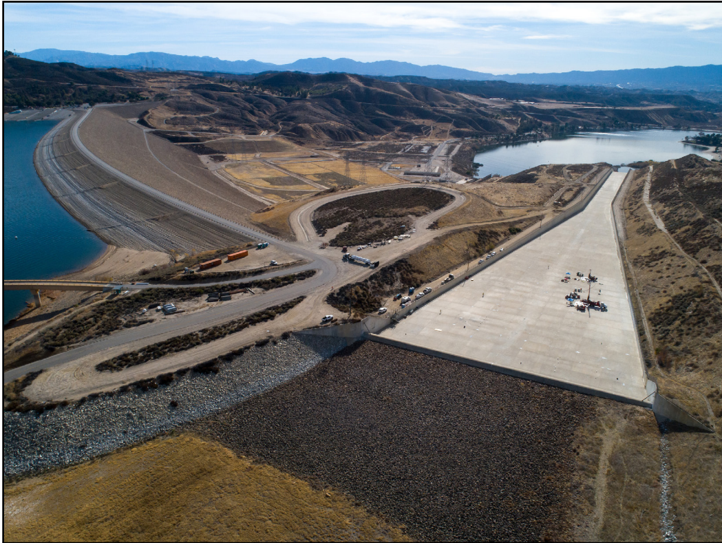
A drone view of the work being conducted by DWR and their contractors as part of a scheduled subterranean evaluation by drilling through the concrete surface on the State Water Project's Castaic Dam emergency spillway in Los Angeles County. Castaic Lagoon can be seen at the bottom of the spillway. Photo by Kelly M. Grow/DWR.
