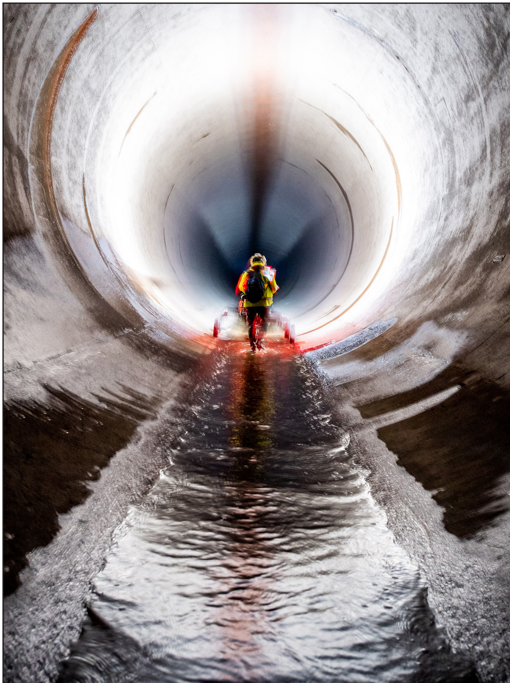
DWR contractors use three-dimensional terrestrial LiDAR (laser scanning) to inspect and survey the Carley V. Porter tunnel, which is 20 feet in diameter and runs more than 25,000 feet across the Tehachapi Mountains in Kern County. Source: Department of Water Resources
