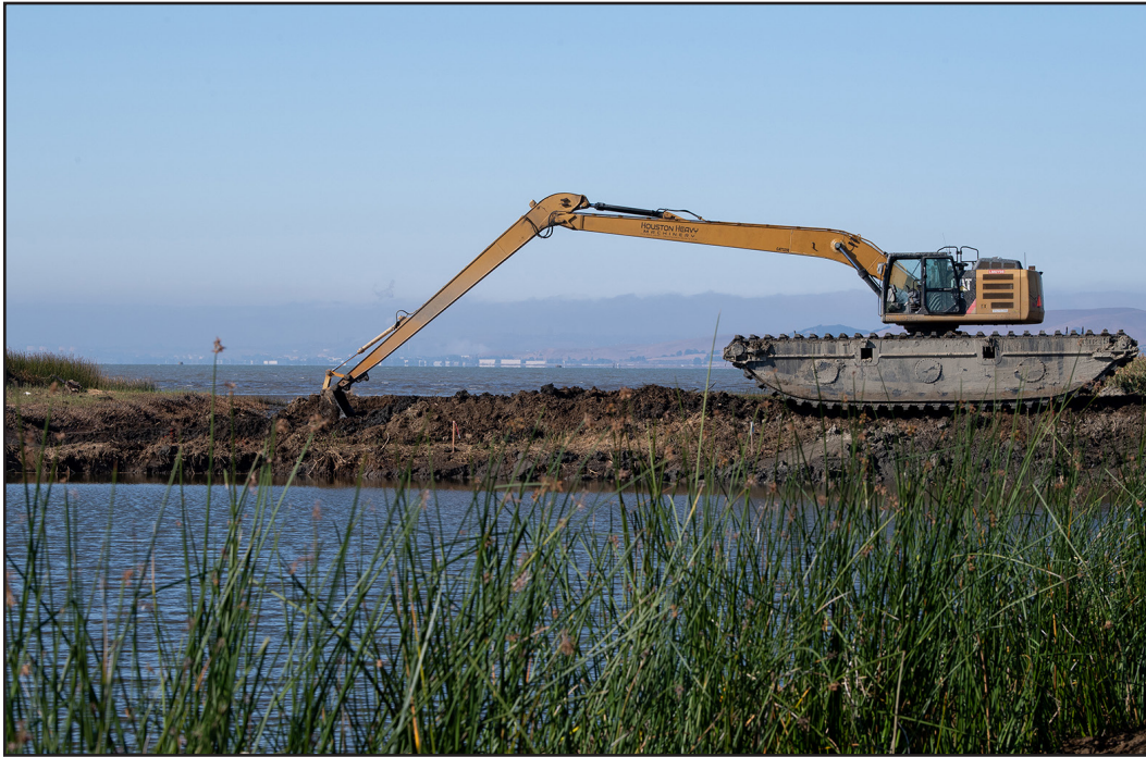
An excavator breaches a levee for the Tule Red Tidal Restoration Project, the first restoration project to break ground in compliance with the U.S. Fish and Wildlife mandate for 8,000 acres of tidal habitat to protect threatened or endangered species. The breach allowed brackish tidewaters to return to more than 400 acres of habitat for Delta smelt, longfin smelt, and Chinook salmon. Source: Department of Water Resources
