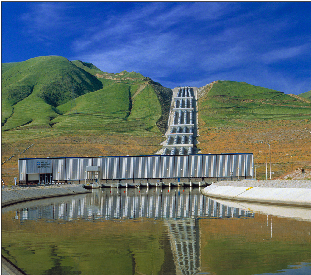
The Ira J. Chrisman Wind Gap Pumping Plant, located just west of Interstate Highway 5 in Kern County. The pumping plant with four discharge lines provides the third in a series of lifts culminating at the A.D. Edmonston Pumping Plant to move the water across the Tehachapi Mountains. Source: Department of Water Resources
