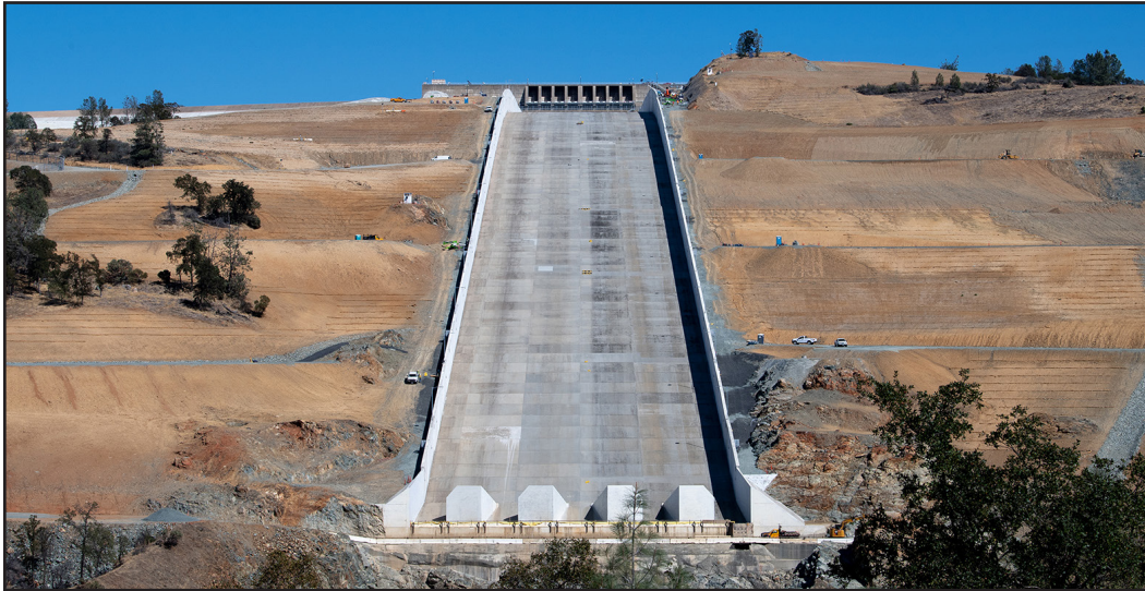
A view of the Lake Oroville main spillway as rehabilitation work continues on the hillsides including grading and erosion control measures, and gravel-lined drainage at the Butte County site.
