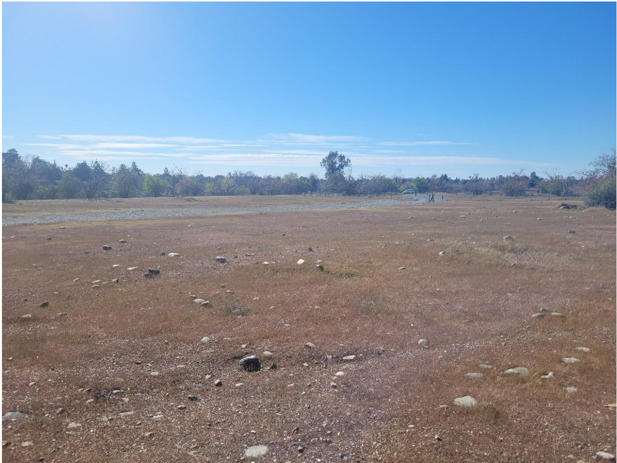
Photo 12 Staging Area 3, looking southwest (February 18, 2022)
