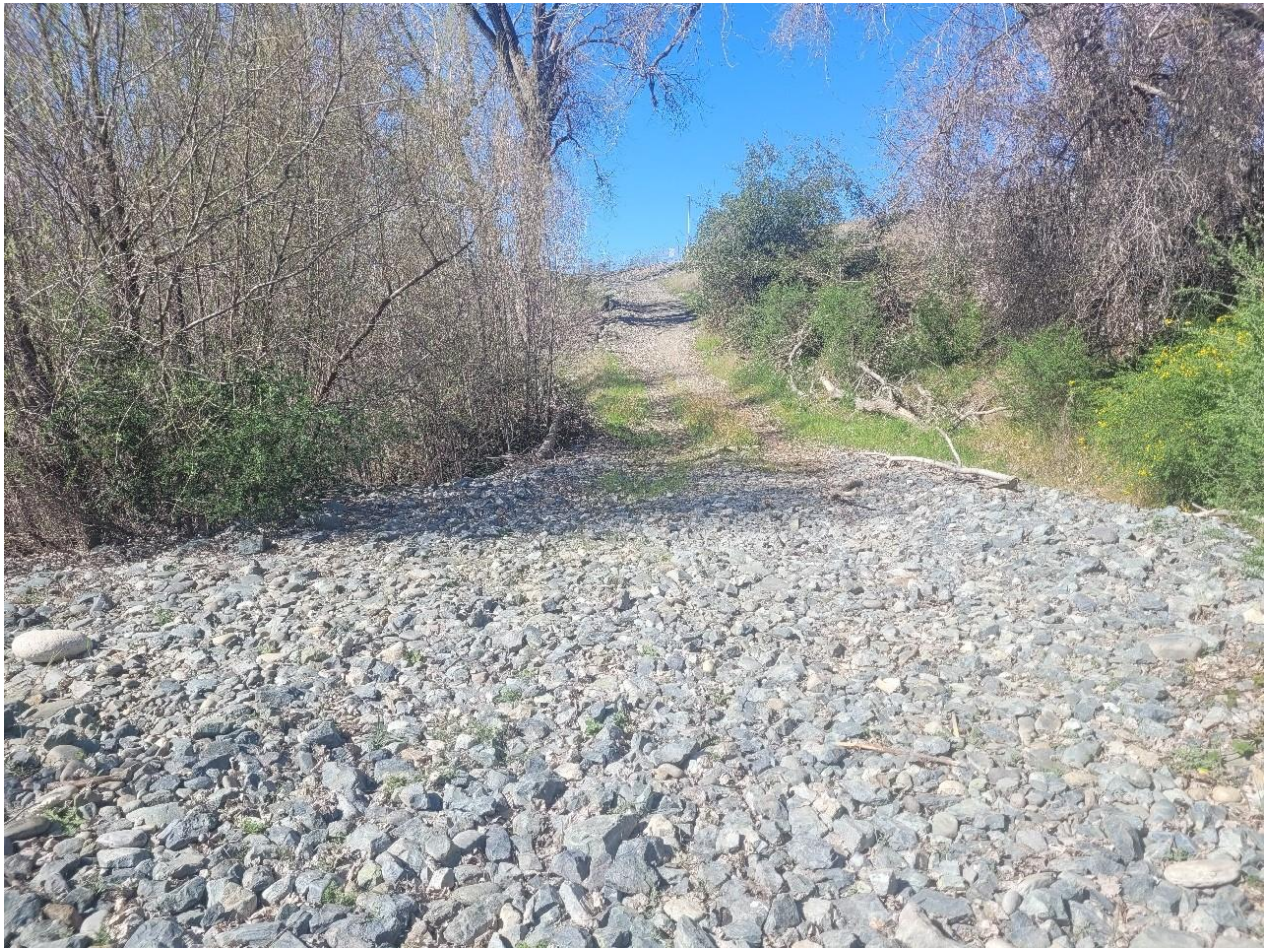
Photo 5 Terrestrial access route Alternative 1 (segment 1B), looking west (February 18, 2022)
