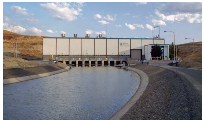
Photo: Las Perillas Pumping Plant
