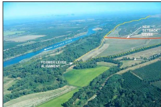
Bear River Levee Setback Project constructed by TRLIA in 2005-06
