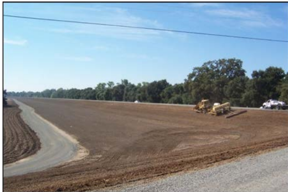
New levee construction at Natomas
