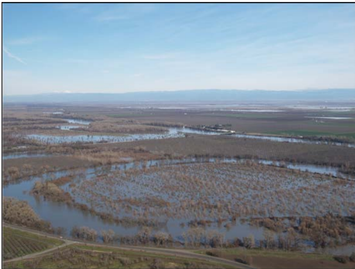
Setback levee at Butte City
