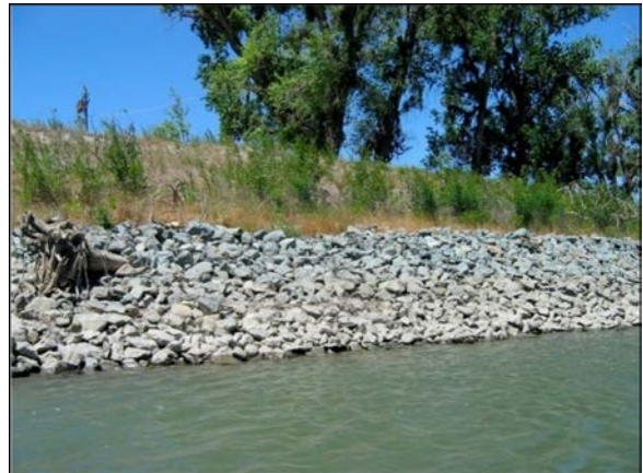
Bank revetment along the Sacramento River
