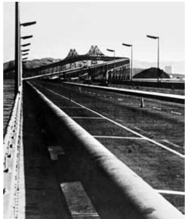
The emergency pipeline constructed across the San Rafael Bridge to bring water to southern Marin County. (see following page)
