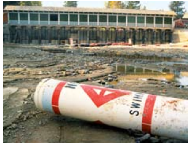
Lake Tahoe Dam is operated by the U.S. Bureau of Reclamation as part of its Newlands Project to supply water for uses in Nevada. The upper 6.1 feet of Lake Tahoe amounts to a usable storage capacity of 744,600 acre-feet (AF).
